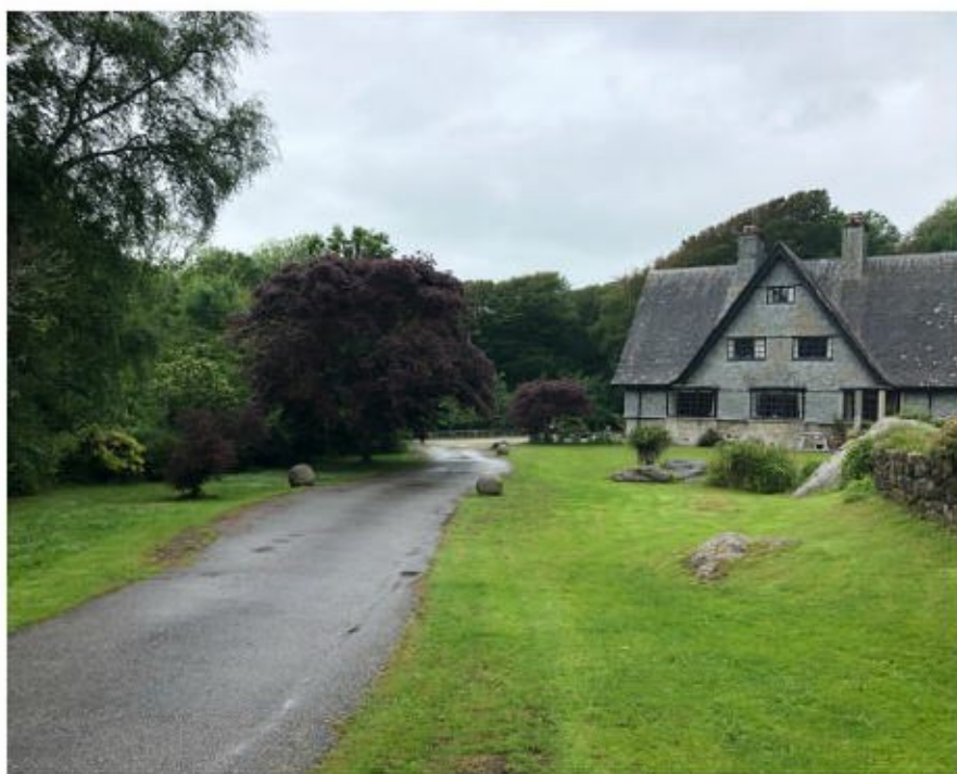
Figure 1 – South elevation of Trevelloe House from drive
