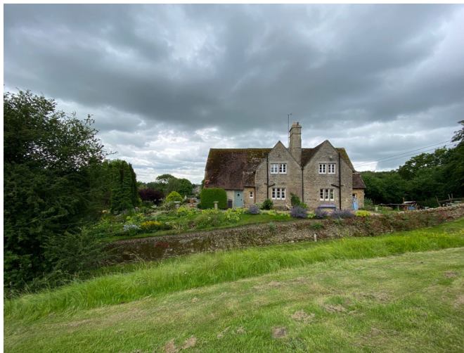
Existing north elevation – Large roof scape on Bradstone addition added to the East.
