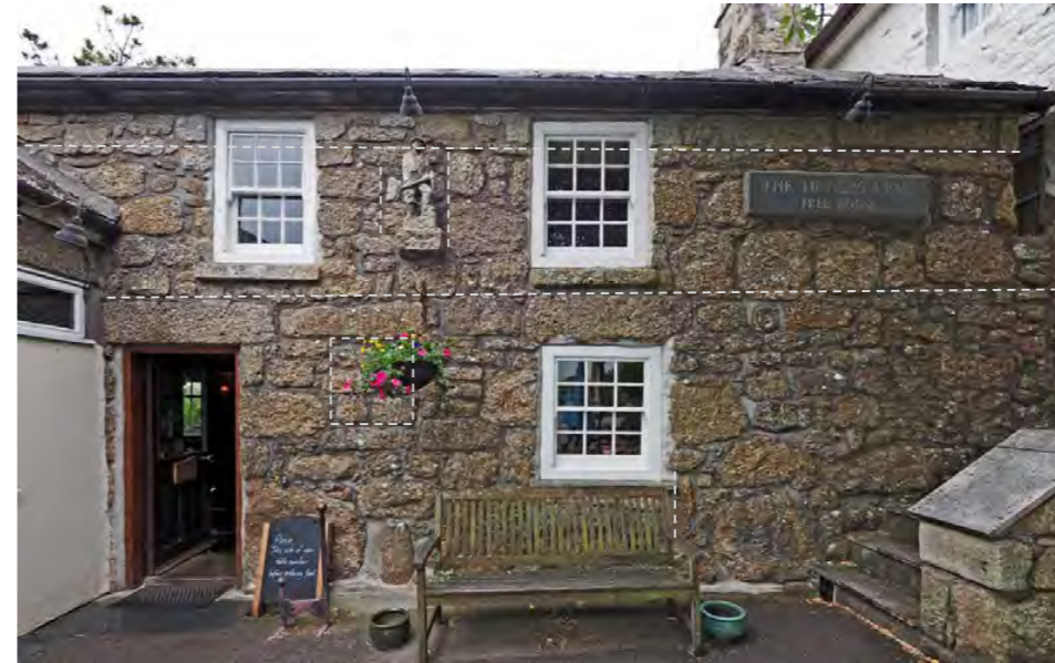
Fig 8: Front wall of original building annotated to show anomalies including: former probable window opening left of centre; re-facing, rebuilding or remodelling of much of first-floor stonework, and original probable eaves level at top
