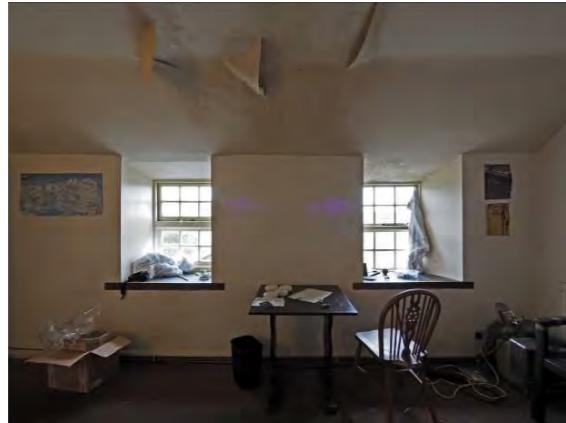
Fig 44: Sitting room SW wall
