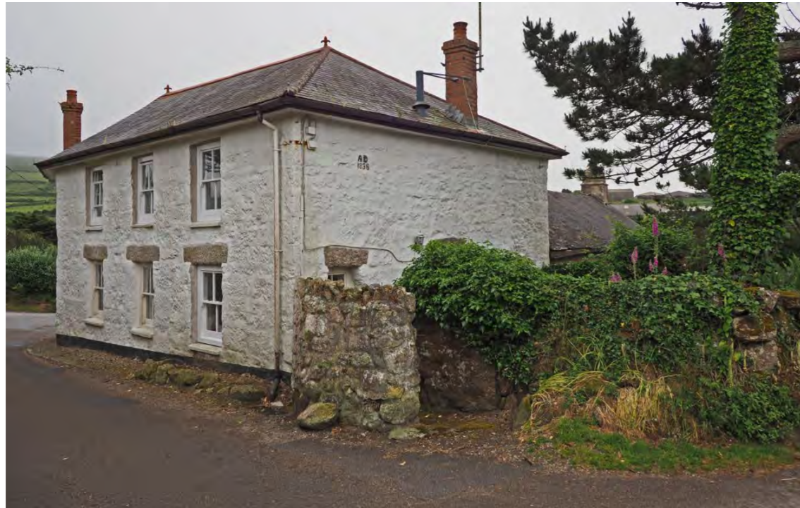
Fig 9: 'Bos Cres' and Tinners from north: note 1838 inscription and reused medieval cross shaft over end window
