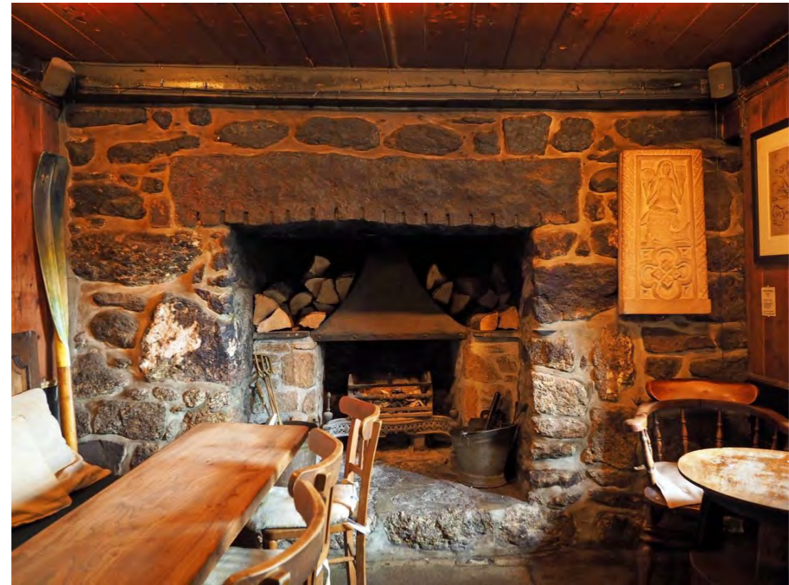
Fig 19: NE fireplace clearly rebuilt in the C19 including granite lintel with drill holes of post 1800 type; traces of limewash indicate former decorative inner wall finish
