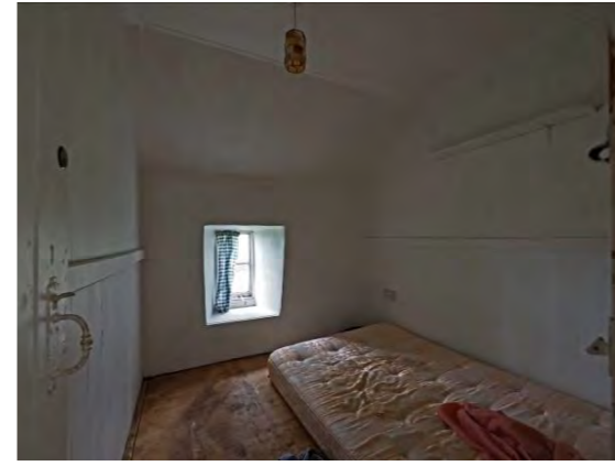
Fig 50: Central Bedroom from south (lit by former stair window)
