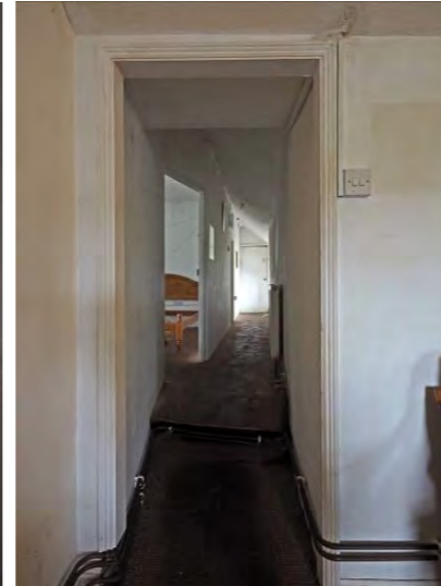
Fig 47: Doorway from Sitting Room to first-floor passage
