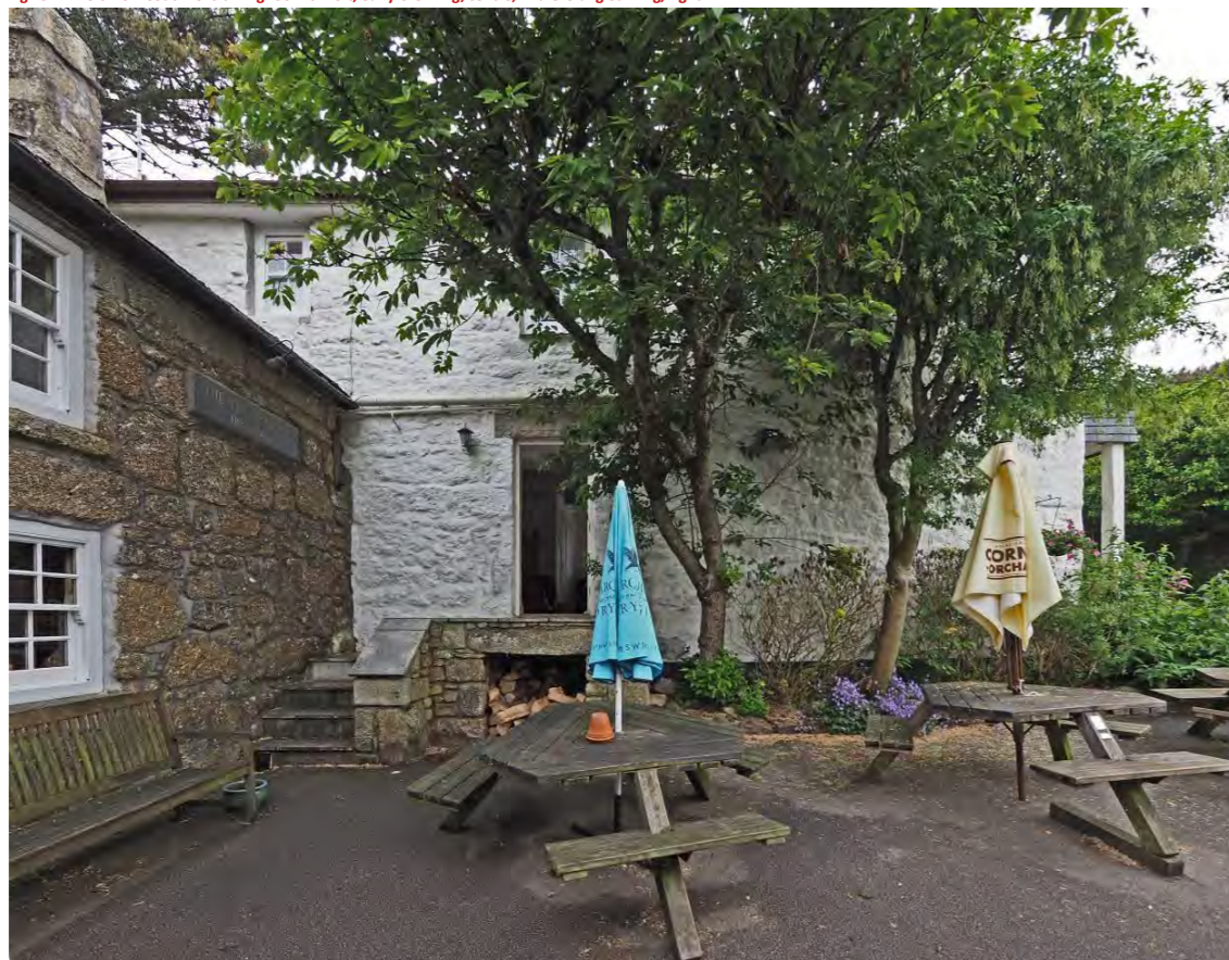
Fig 14: 'Bos Cres' from SW showing functional relationship with the SE courtyard of Tinners
