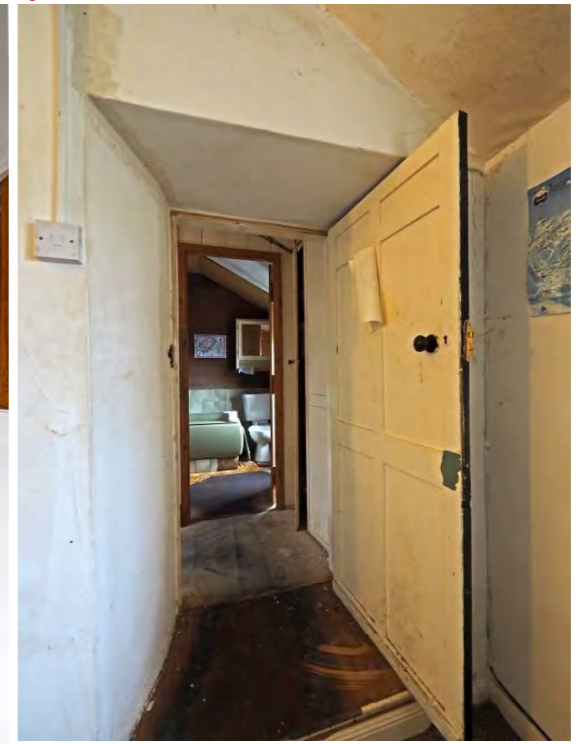
Fig 55: From Sitting Room to Stair Landing and Bathroom
