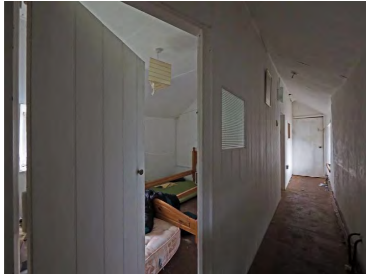
Fig 46: First floor over original building from south
