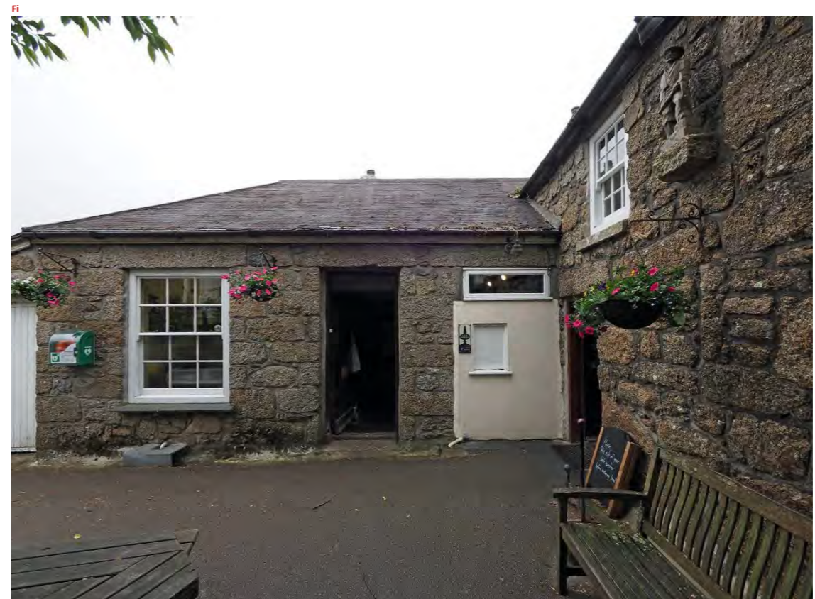
Fig 15: Tinners late C19 or early C20 extension, left and centre, now containing kitchen and serving bar
