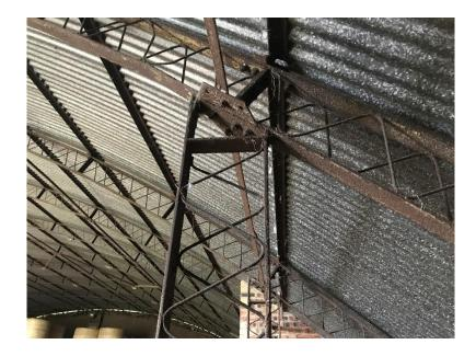
The gables to the building are formed with 190mm x 80mm vertical steel channel stanchions arranged vertically at 4.5m centres and secured to the trusses. The gables are similarly clad with corrugated galvanised sheeting with painted finish secured to with U bolts in a similar fashion to the roof.
