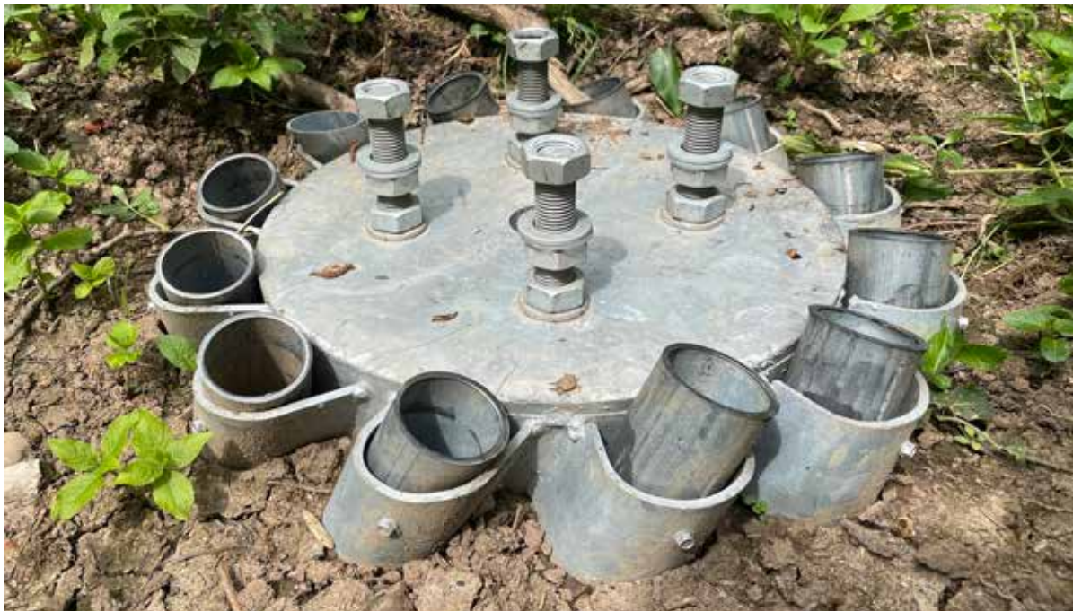
3. ROOT PILE CAP DETAIL
