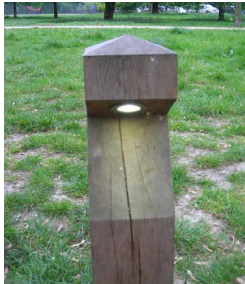
DIRECTIONAL SHIELDED LIGHTING EXAMPLE FOR ACCESS
