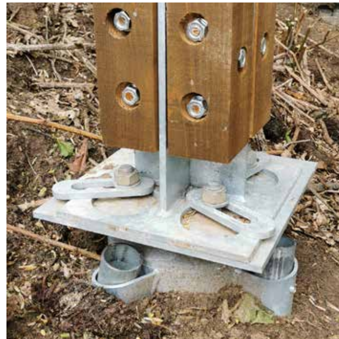
4. ROOT PILE CAP WITH POST ANCHOR
