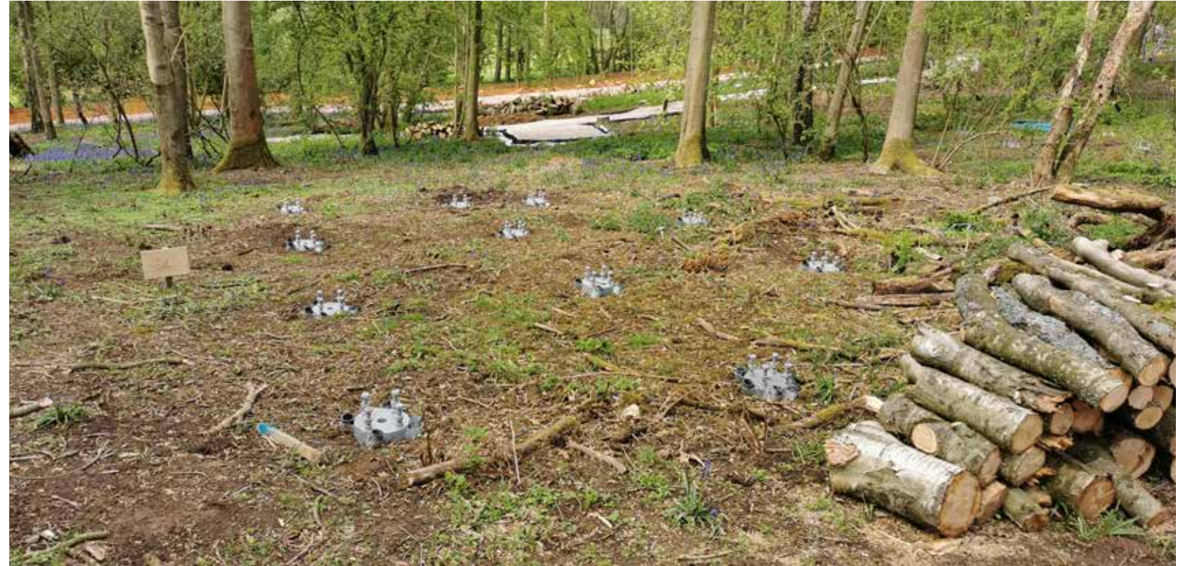
2. ROOT PILES INSTALLED
