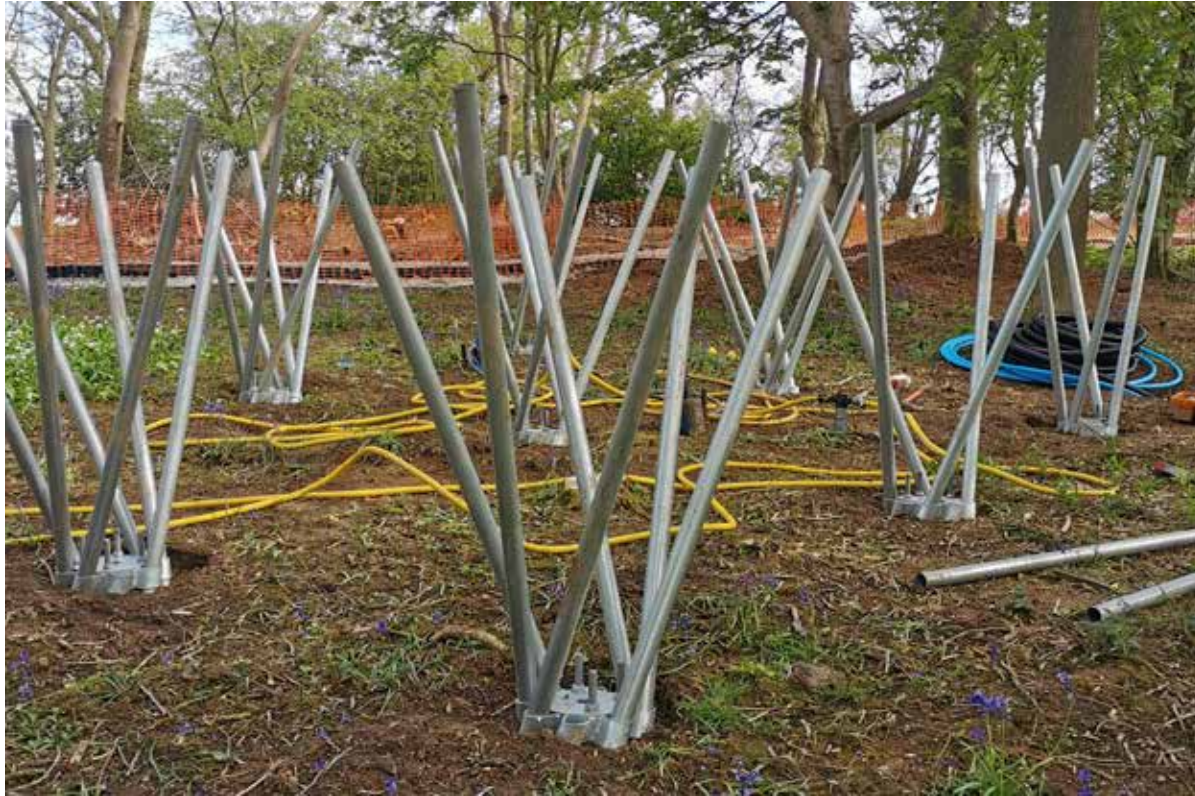
1. ROOT PILES SET OUT FOR INSTALLATION
