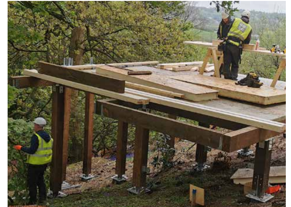
5. BUILDING FRAME ERECTED ON PILE CAPS
