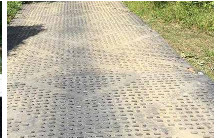
IMAGE B - TEMPORARY GROUND MATS
