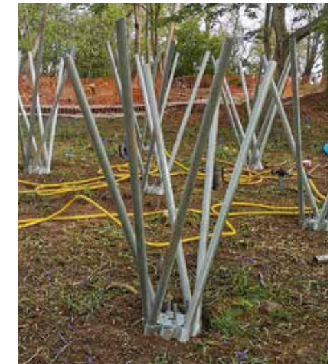
RAPID ROOT PILE
