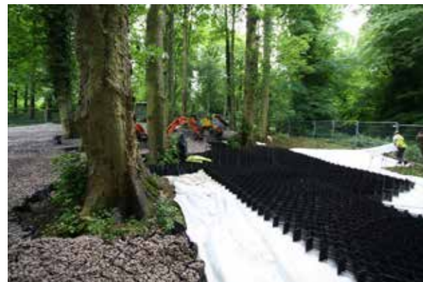
Ground protection measures mitigate damage to trees
