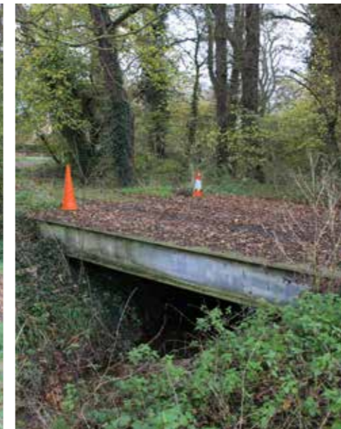
Existing bridge over stream
