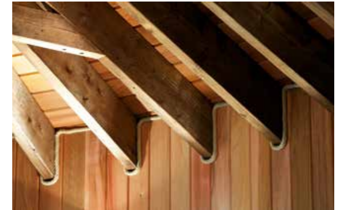
3. Rope detail of internal junction
