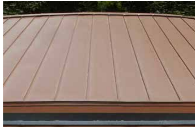
1. Copper standing seam roof
