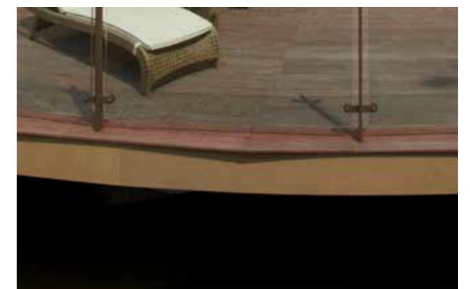
9. Detail of decking and substructure
