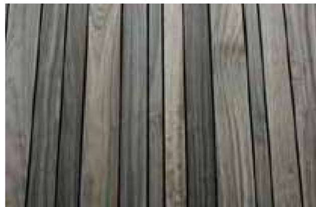
4. Varied widths of vertical Cedar cladding
