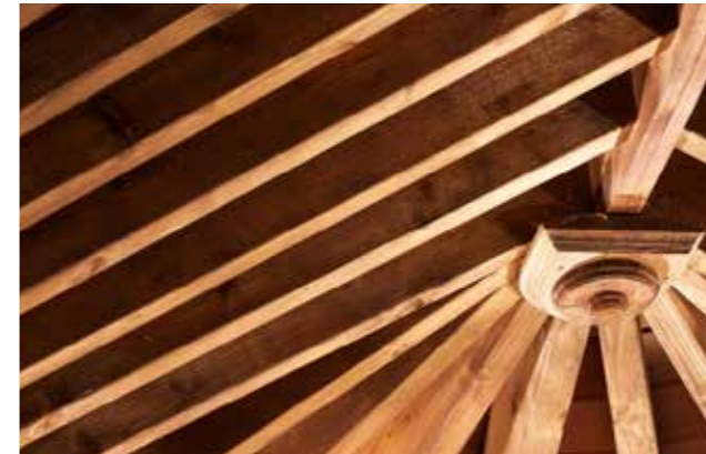
2. Softwood timber rafters with Cedar sarking boards
