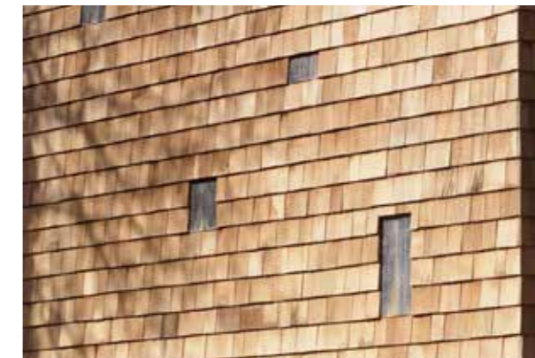
Bat and bird roosts built into wall
