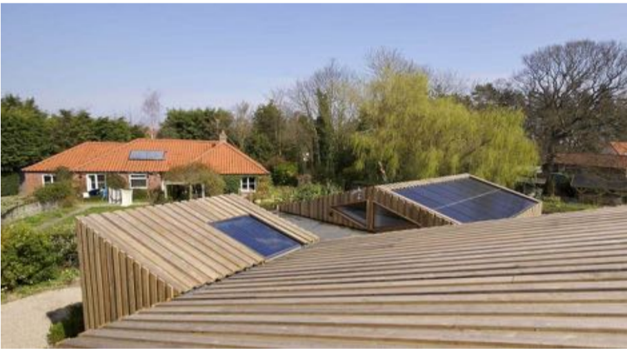
integrated solar thermal and pv roof panels
