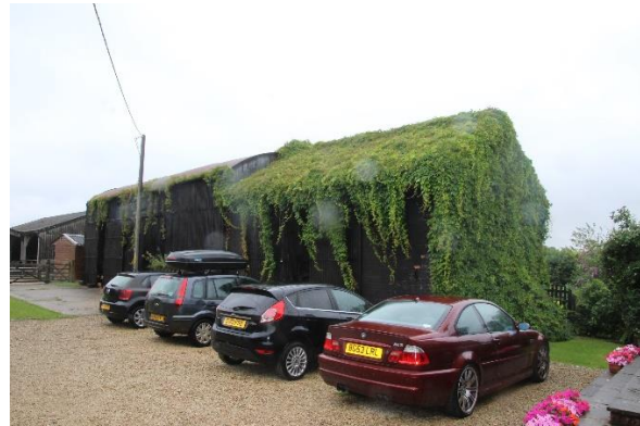
2. Pitchers Barn from the north-west
