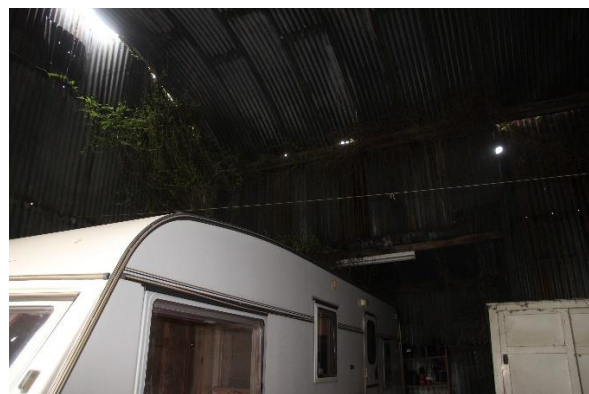
6. Internal space of Dutch barn looking south-west
