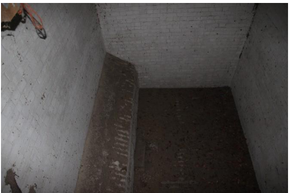
8. Internal view of one of the silos from above
