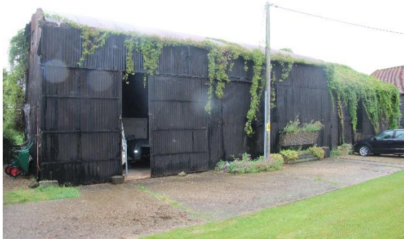
1. Pitchers barn from the north-east
