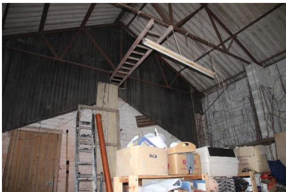
5. Internal space of western barn looking east
