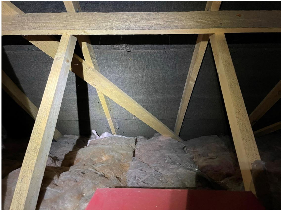
4. Wooden rafters with bituminous felt.
