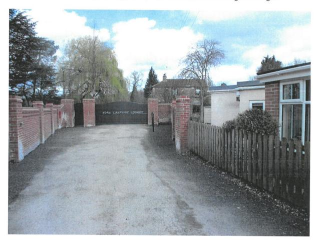
4.2 The walls are of blockwork and red brick construction. At their highest point the brick columns are 2.55m high. The main body of the wall is 1.75m high, interspersed with 2.05m high columns. The gate is of close boarded timber construction set on a metal frame with decorative metal railings on top. The gate opens by way of a sliding mechanism.
