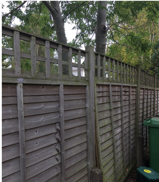
Photoview 1 - note displacement of fence panel.
