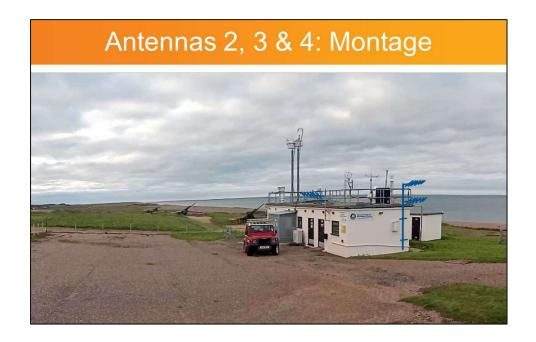
The fixings for the antenna will be steel scaffold poles and mounting brackets. Antenna 1 will be fixed to the metal stairs as shown below extending 1m horizontally from the stairs and a further 2m (the length of the antenna) parallel to the wall.
