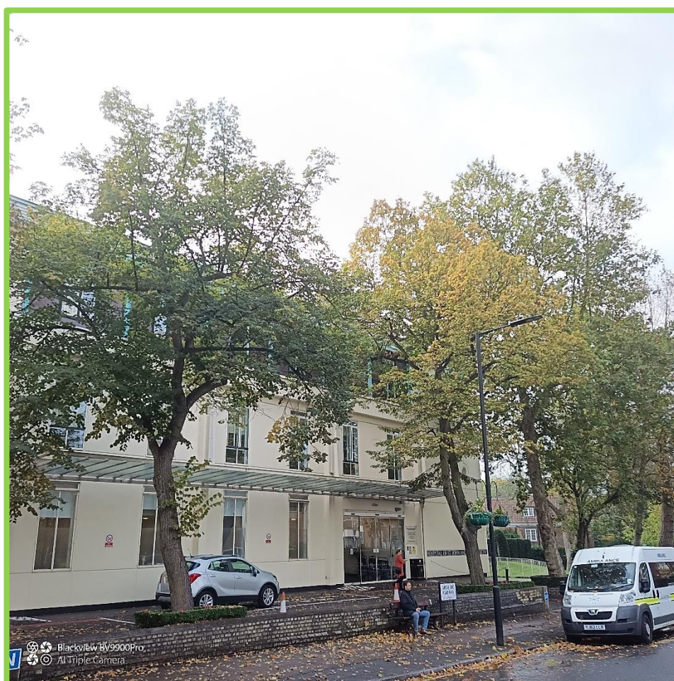
TREES TO THE SITE FRONTAGE AND MAIN ENTRANCE TO THE HOSPITAL OF ST JOHN AND ST. ELIZABETH
