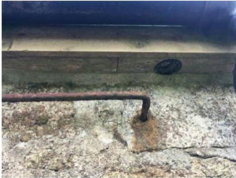
Photograph 3. Tightly fitted soffit box.
