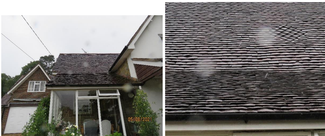
Figures 11 & 12. The catslide roof on southern elevation where a new two storey extension is proposed. Example of general tile gaps in this area.
