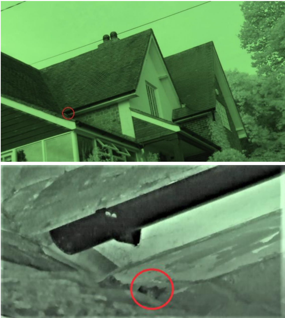
Figure 4. Showing Brown Long-eared bat emergence point at southern elevation. The roost entrance is a small mortar gap at the junction between the main roof valley at a point where it meets the cat-slide roof and abutting the original stone walls, under the soffit and gutter. In the close up, a Brown Long-eared bat can be seen in the roost entrance at point of emergence.
