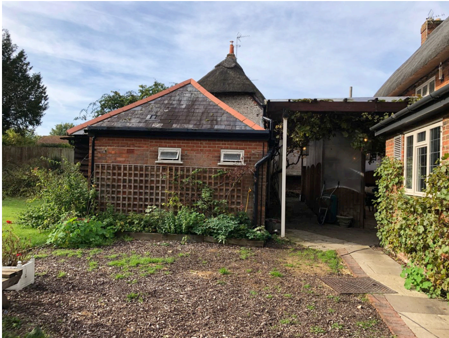
Rear Covered area to be replaced
