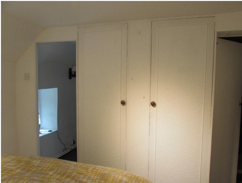
Figure 3- cupboards and wall to be removed.
