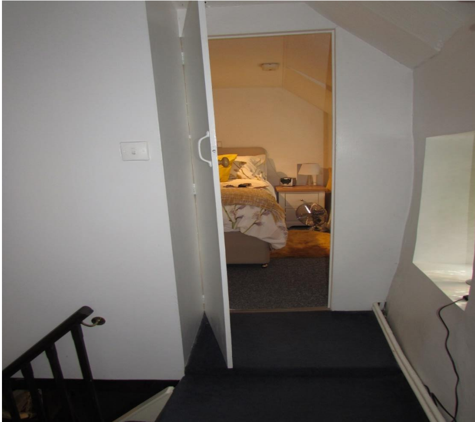
Figure 4 - cupboards, and wall to be removed, view from landing.
