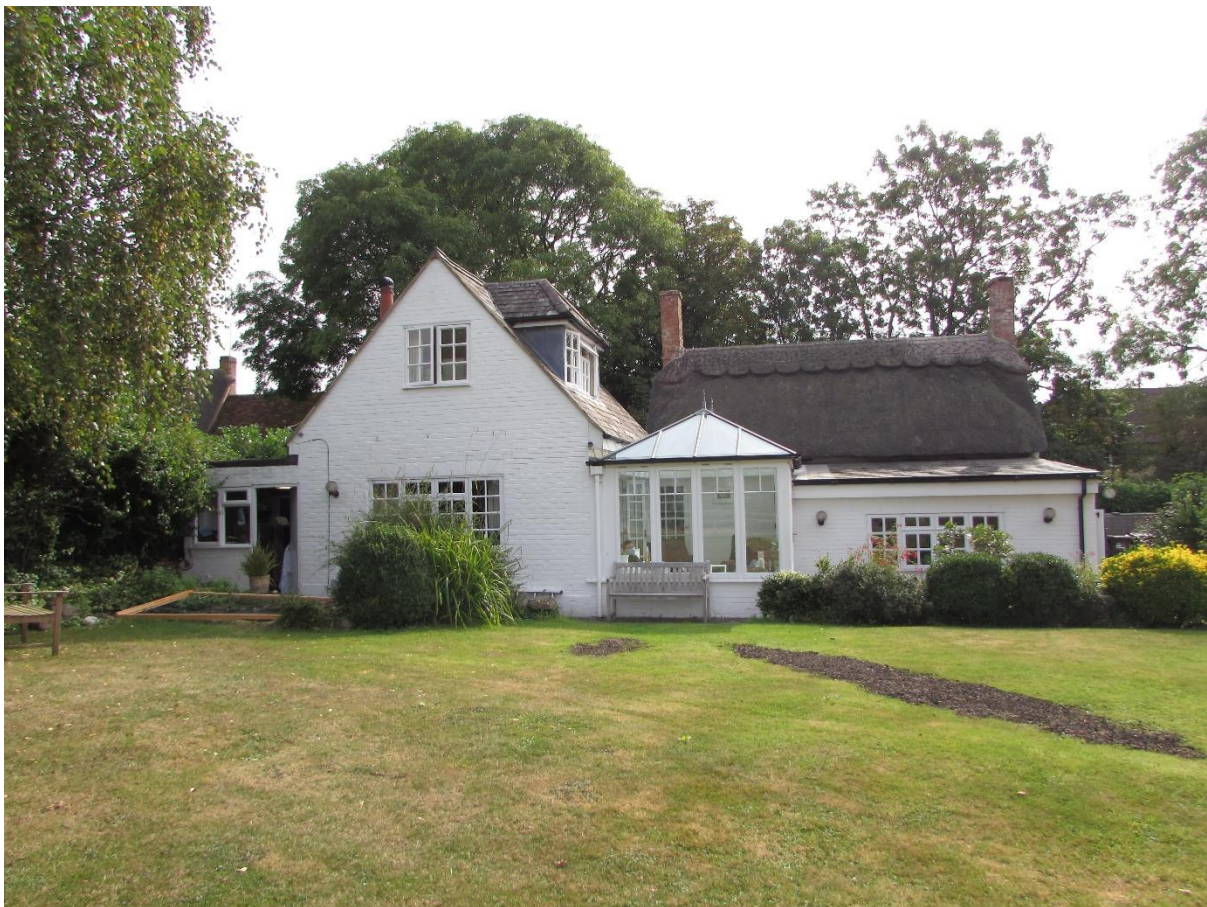
Figure 8 – Rear view of property
