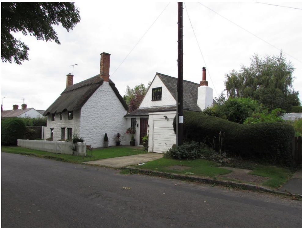
Figure 5- showing garage and chimney stack to be demolished.
