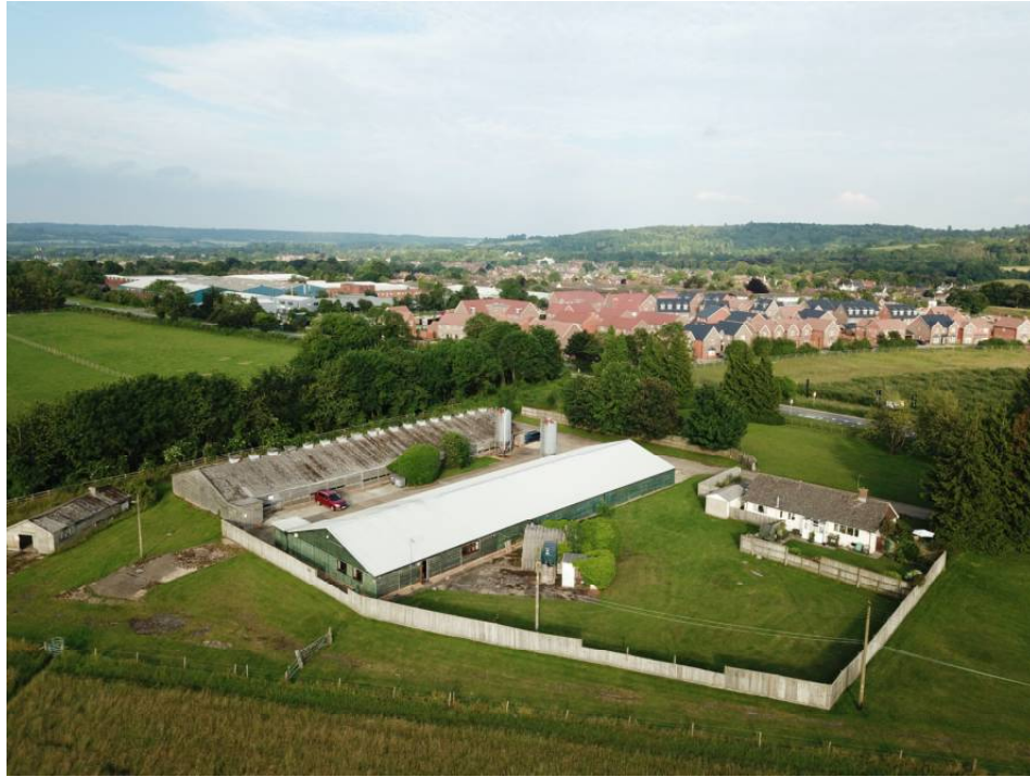
Image 4 – Existing buildings, fencing and planting on the Site
