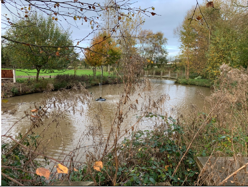
Pond with vertical sides, poor water quality, wildfowl present and submersible pump and fountain
