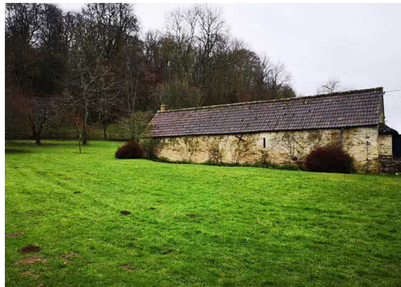
Fig 2 - Rear of current Studio building, facing East
