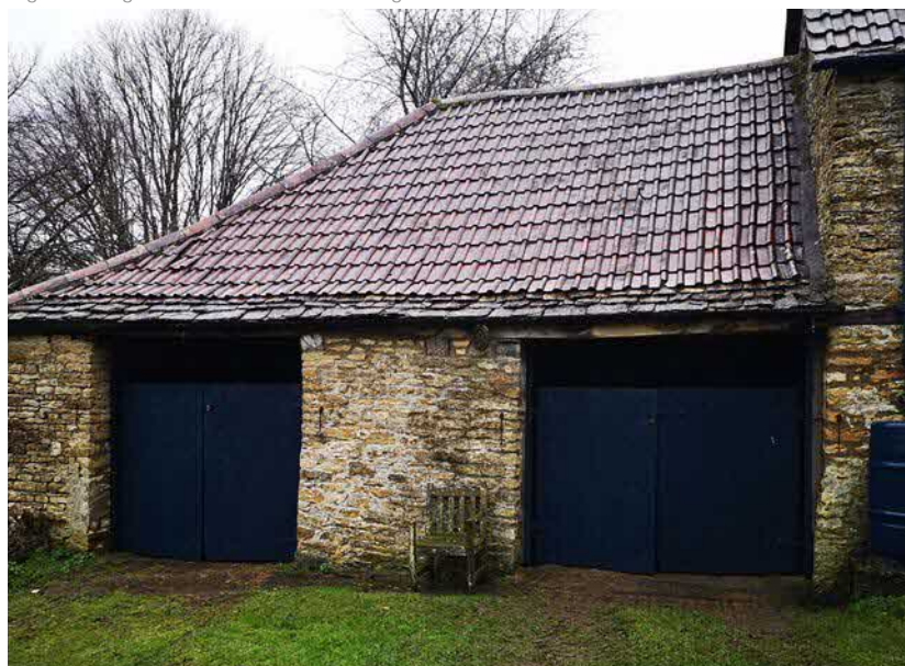
Fig 6 - Former Cart Shed, Front, facing West
