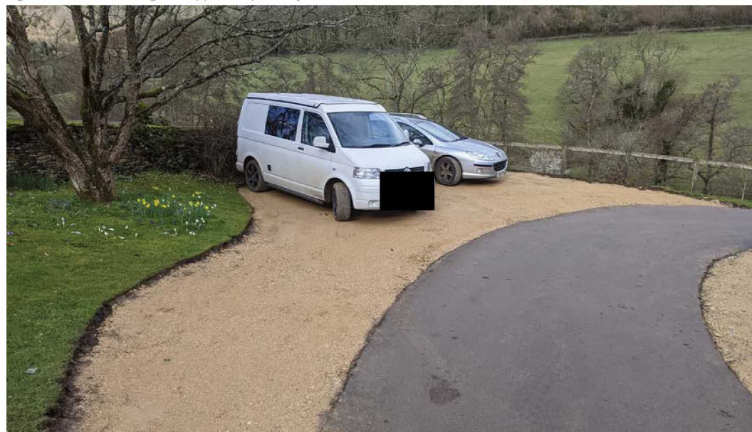
Fig 5 - Lower Car park and drive
