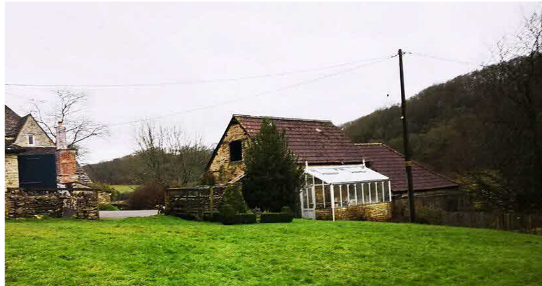
Fig 3 - Former Cart Shed Rear facing East, with existing planning permission to convert into separate accommodation
