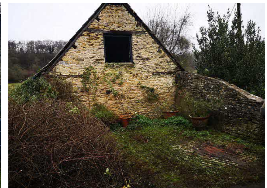
Fig 7 - Former Cart Shed, Side, facing South
