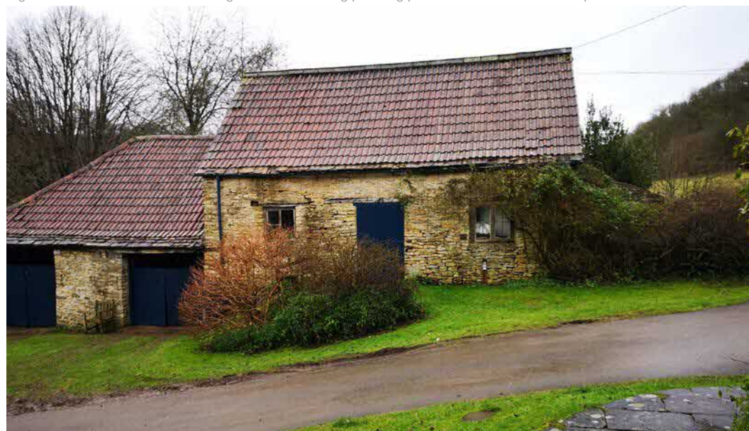
Fig 5 - Former Cart Shed, Front, facing West, with existing planning permission to convert into separate accommodation
