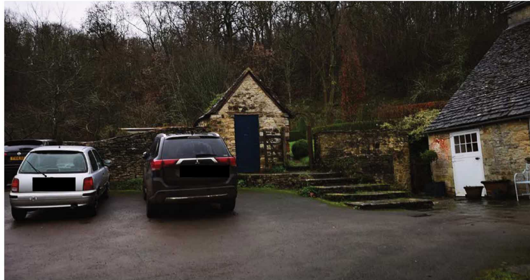
Fig 3 - Small Outbuilding and upper car park adjacent to Kitchen
