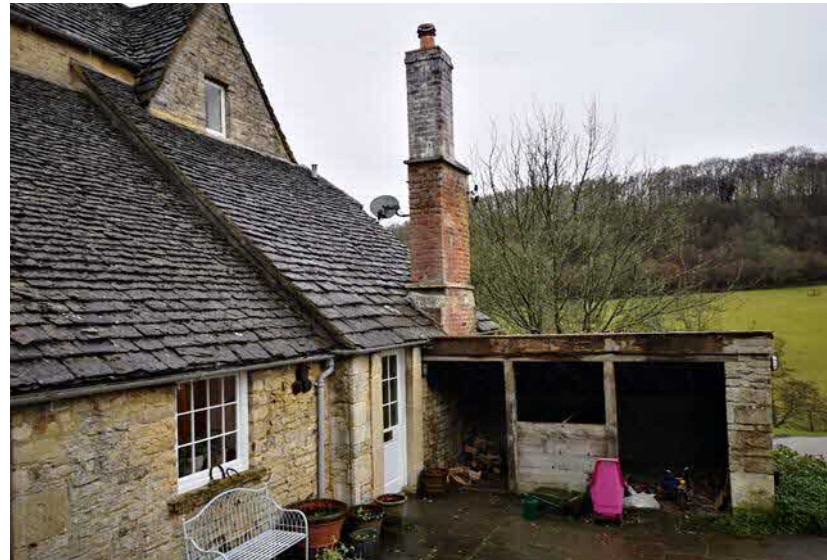
Fig 4 - Lean too Log store and views beyond to the North
