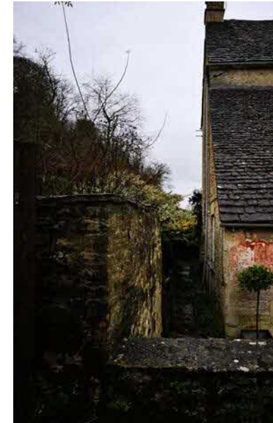
Fig 7 - Access pathway below retaining wall behind Rear wall facing south
