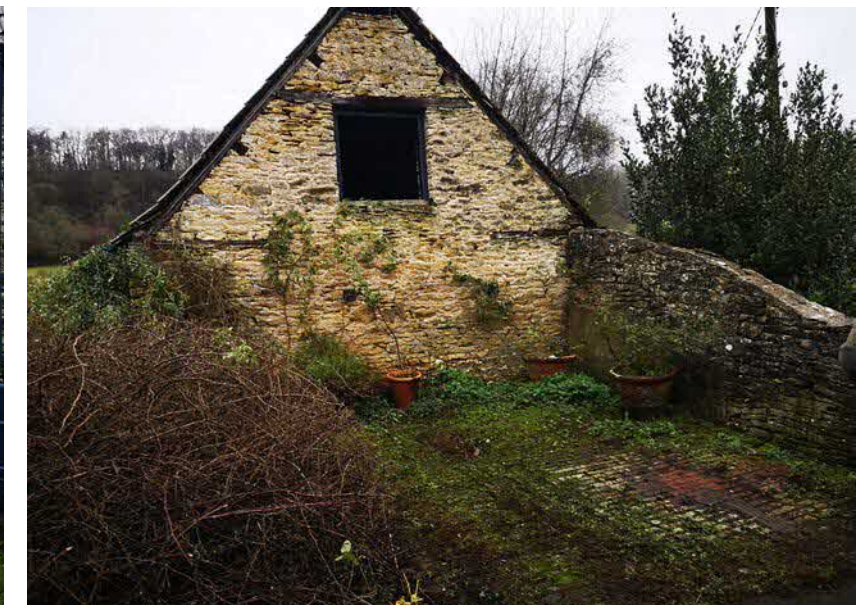
Fig 7 - Former Cart Shed, Side, facing South
