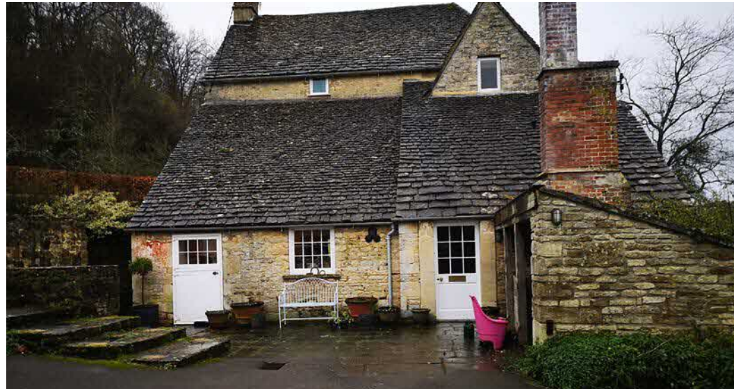
Fig 3 - Lean too Kitchen entrance and back door facing East
