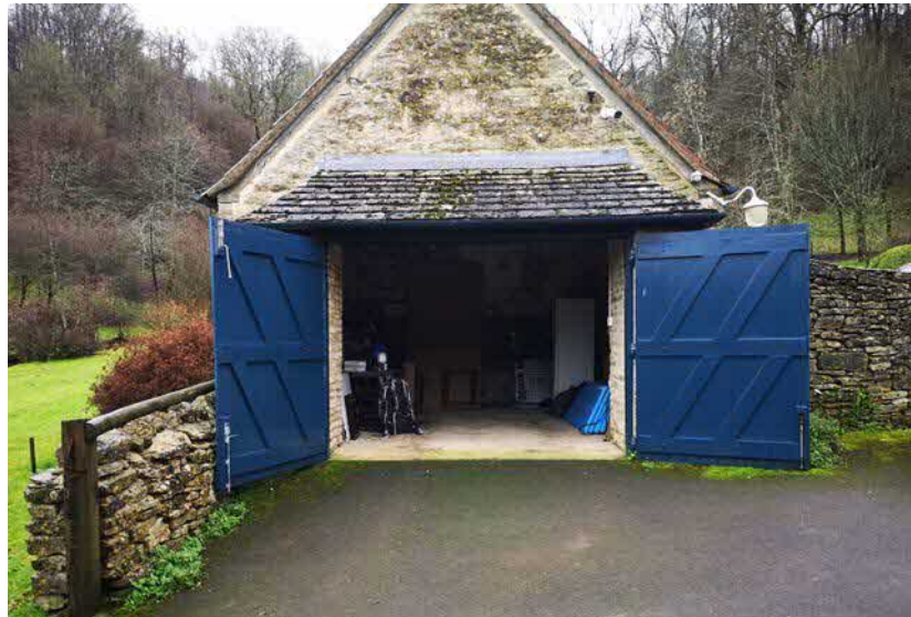
Fig 4 - Garage attached to Studio Building
