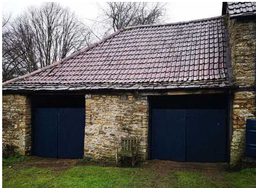
Fig 6 - Former Cart Shed, Front, facing West
