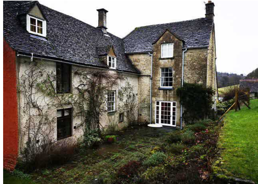
Fig 2 - Rear facade of the farmhouse facing south
