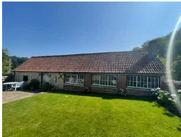
Photograph 1: New lawn and patio area.
