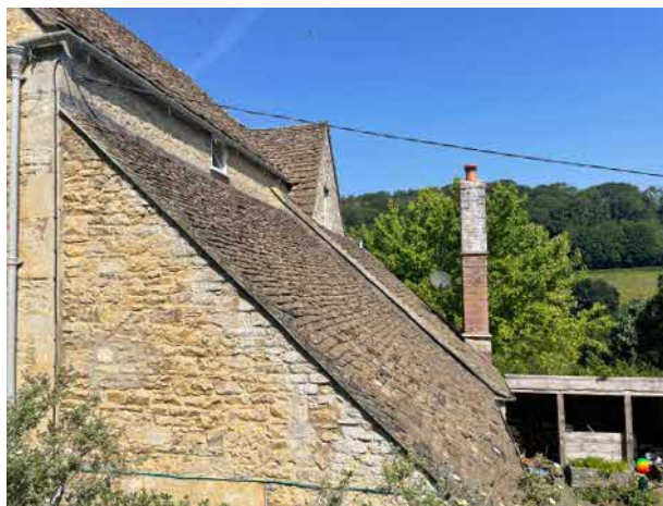
Photograph 5: House – kitchen lean-to roof – south elevation.
