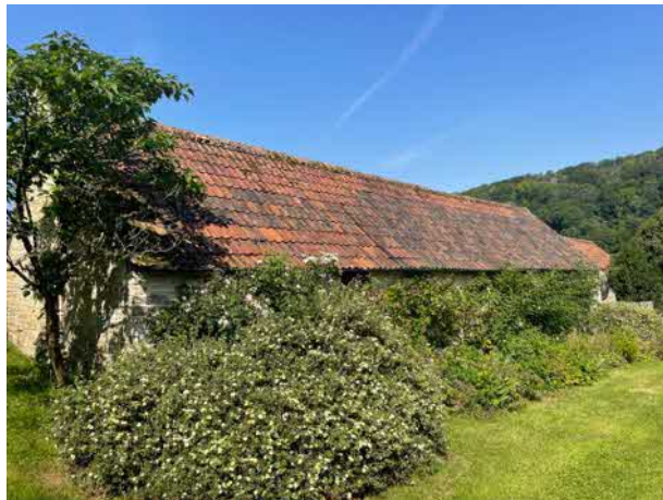
Photograph 9: Annex – east elevation.
