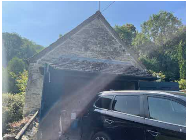
Photograph 10: Annex – north elevation.
