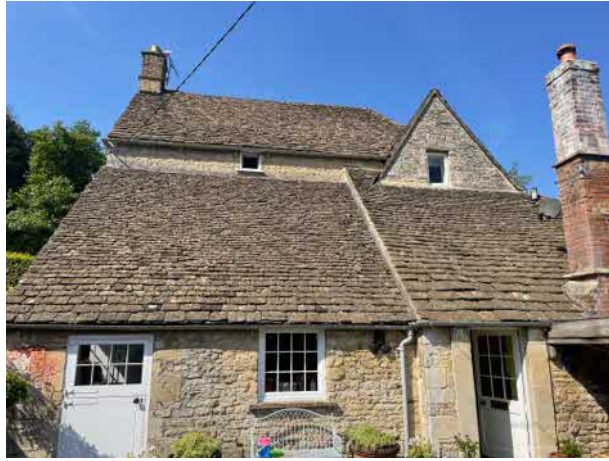
Photograph 4: House – kitchen lean-to roof.
