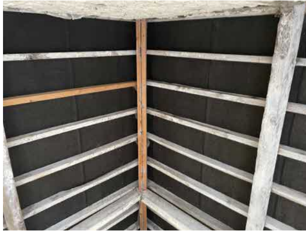
Photograph 12: Annex – garage roof interior.
