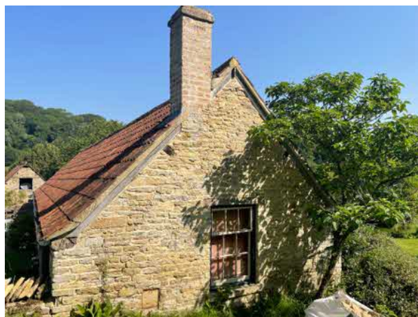
Photograph 8: Annex – south elevation.
