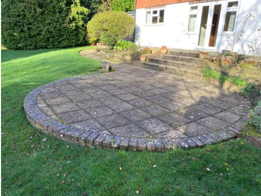
Patio and level change at the rear of the house
