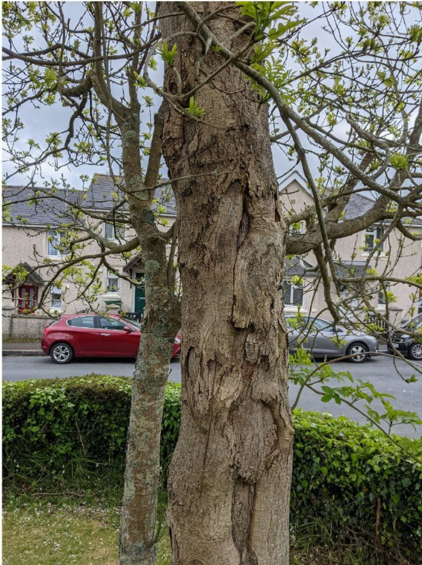
Photograph 6 showing stem damage to ash tree G9.
