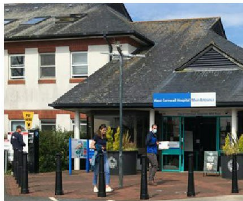
09 - Existing main entrance
