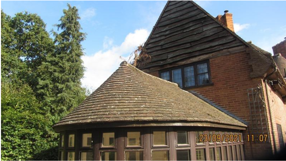
Photo 5: Curve roofed extension
