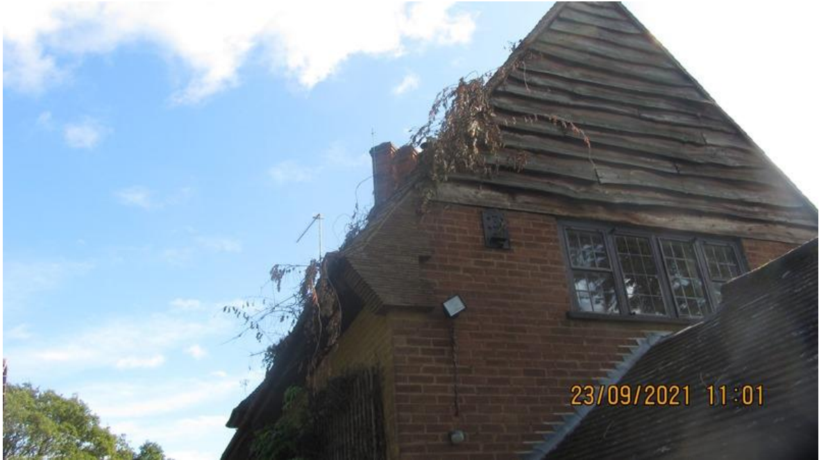
Photo 7: Lifted weatherboarding
