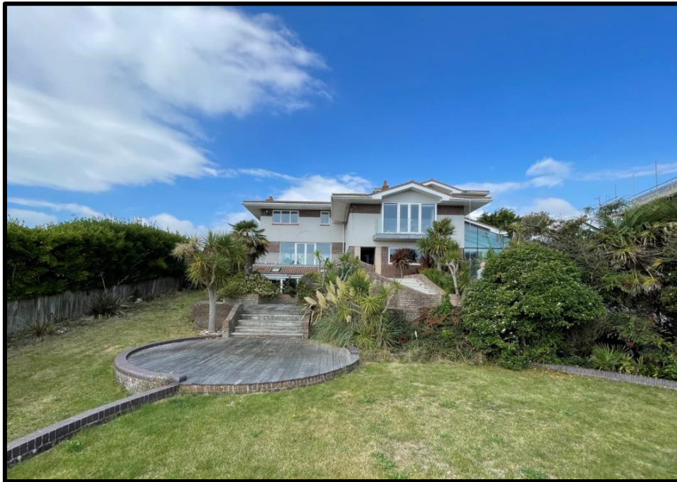
Application property from within front garden
