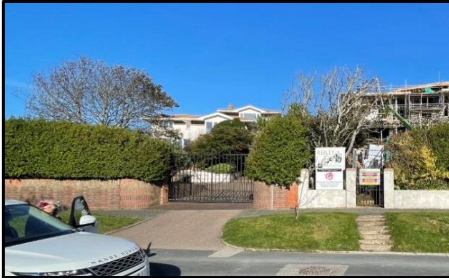
5 Roedean Crescent (7 Roedean Crescent to right)
