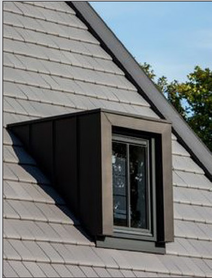
4. Example of metal clad dormer window on slate tile roof of similar proportions and detail.
