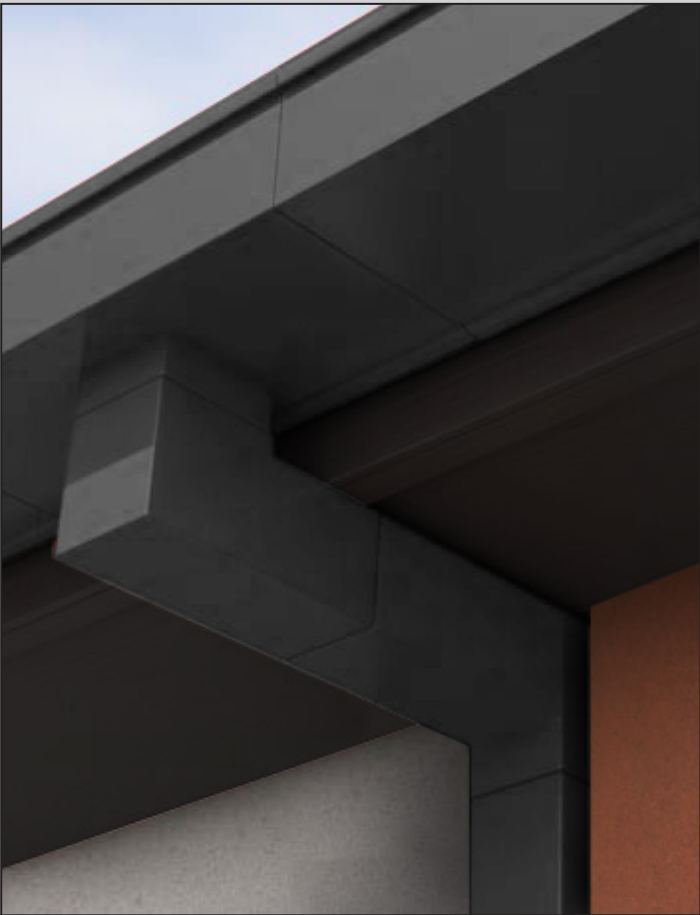
2. Rainwater pipe at the eaves flush with the external render held off by deliberate 25mm shadow gap.
