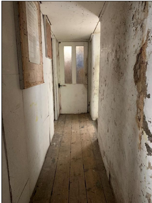
Rear access corridor.
