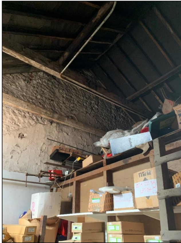
First floor storage
