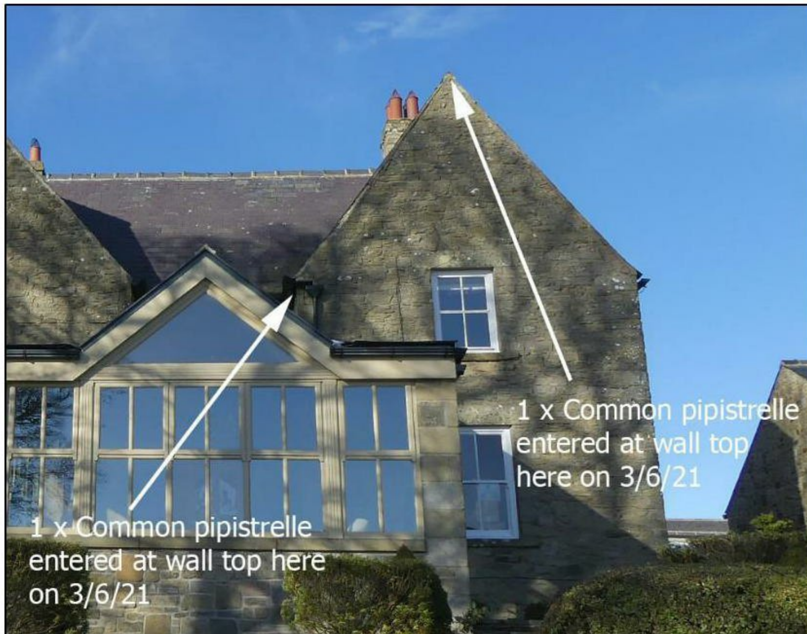
East end of South Elevation of House
