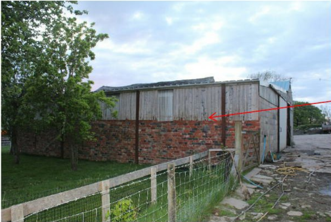
Brick walls and Yorkshire boarding in good condition
