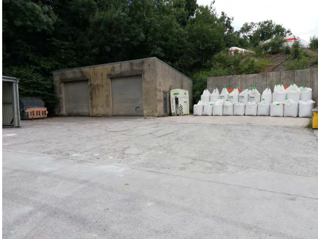
47. Further storage areas, including AdBlue filling point. Garages/stores contain bagging material (plastic/paper). Dumpy bags contain limestone. Looking SW.
