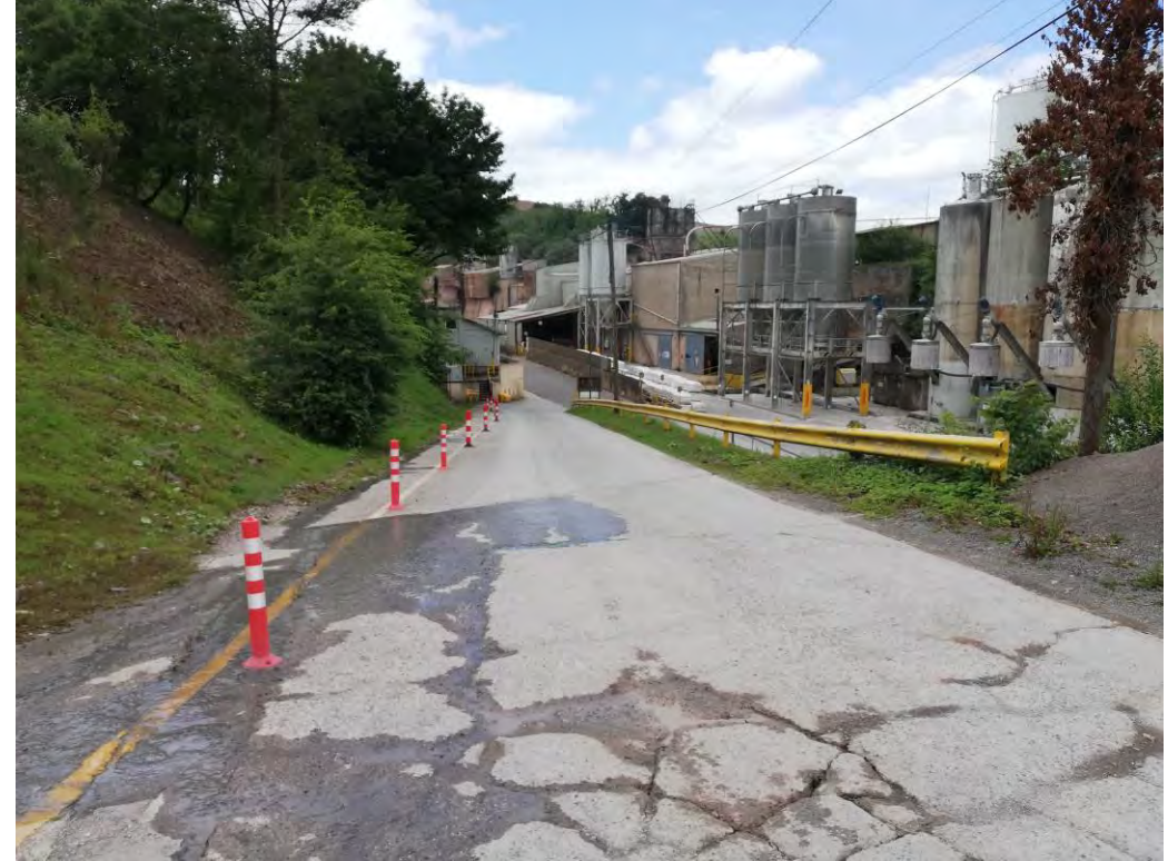
34. Site access road, sloping down to W. LKAB Minerals Ltd limestone/marble crushing plant visible (off-site). Looking NW.
