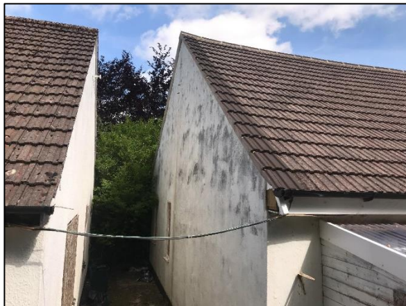
Photo 3 gable end and roof of B1
