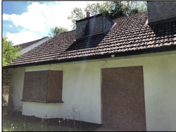
Photo 5 northern elevation of B2
