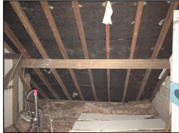
Photo 6 attic void in B2
