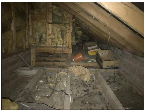
Photo 5 attic void in B1
