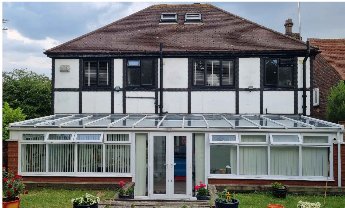
Existing Rear Elevation 3D
