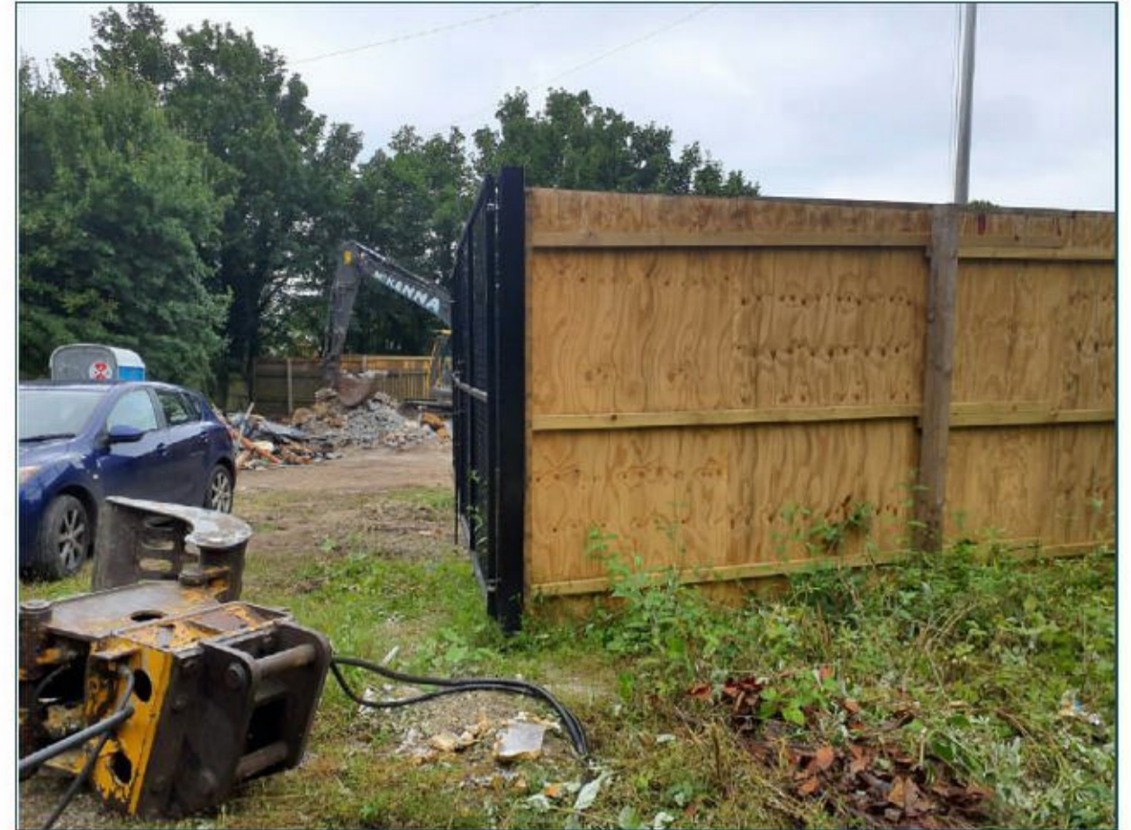
Photograph 2. Shared access into the Site.
