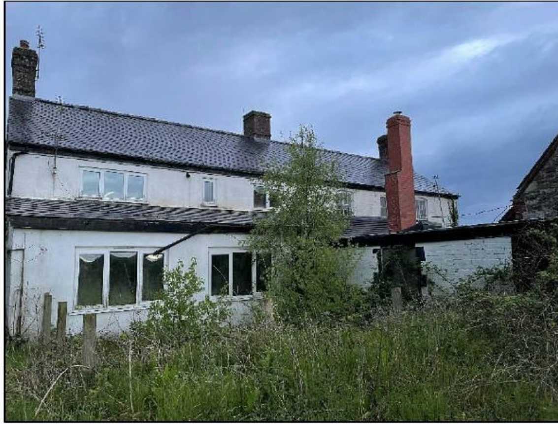
Plate 20. North-eastern elevation of Inn and extension and overgrown garden
