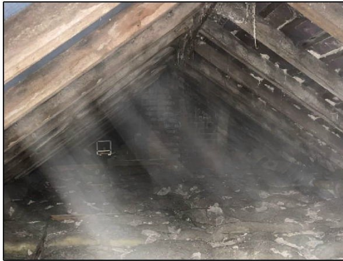
Plate 22. The roof void at the apex of the Inn roof
