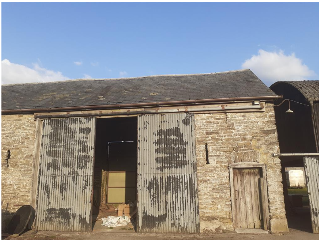
Plate 4: The western elevation of the stone barn.
