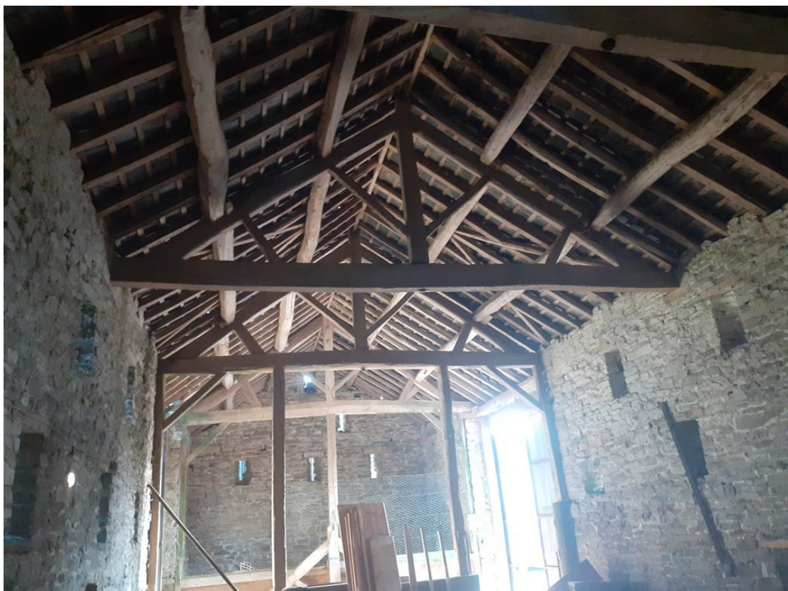
Plate 6: The interior of the stone barn facing southwards.
