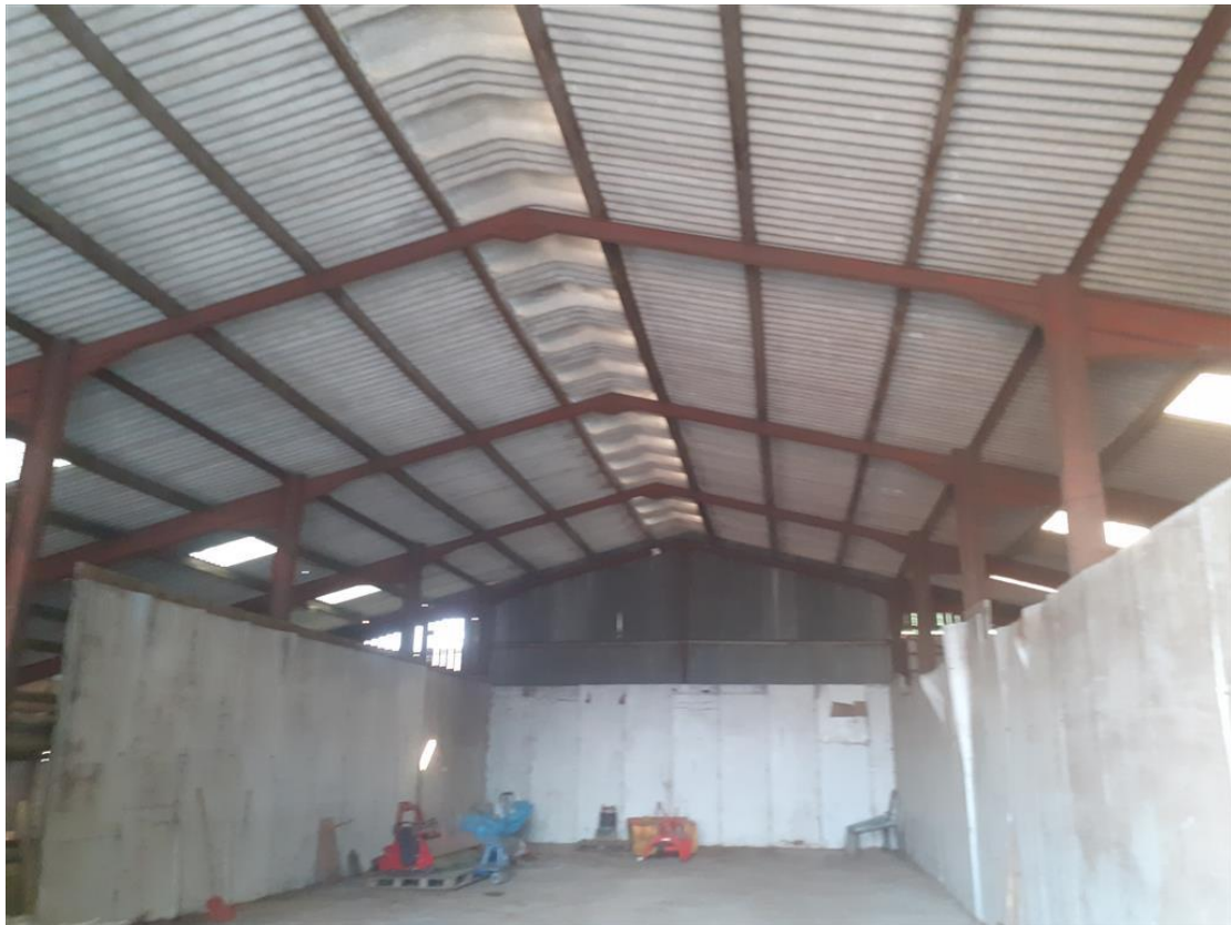
Plate 3: The interior of the main agricultural barn facing southwards.
