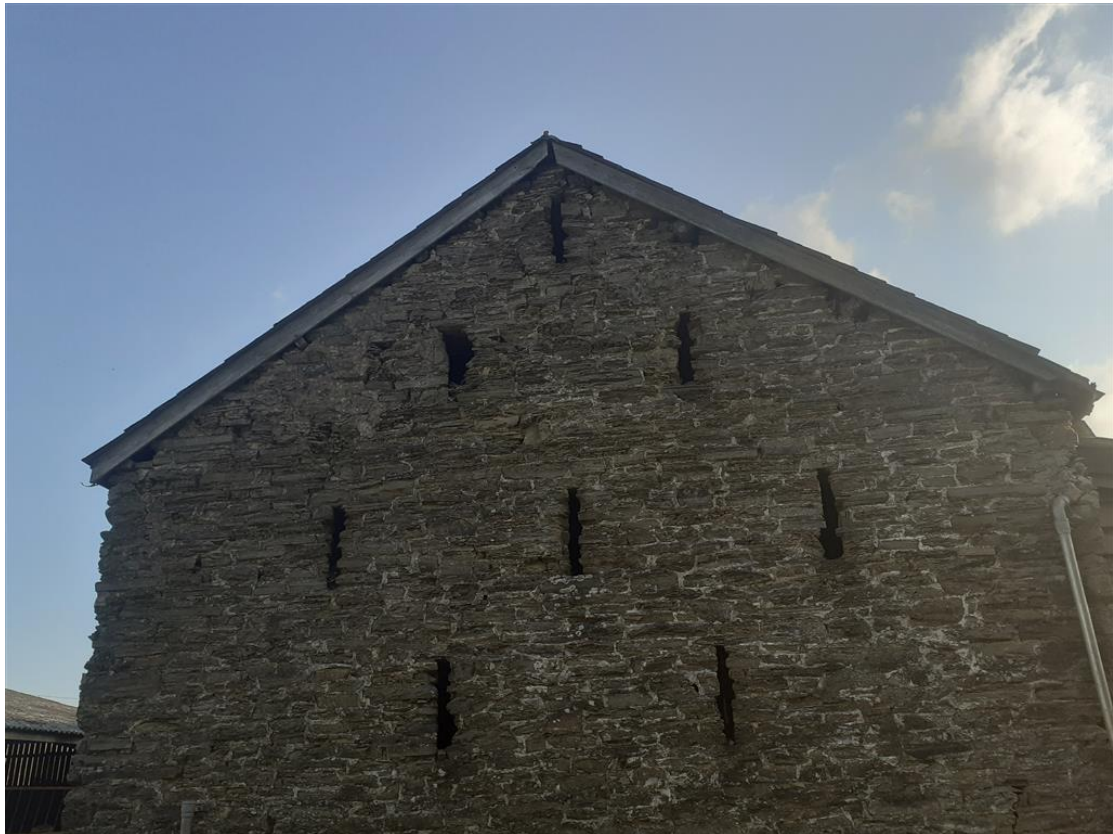
Plate 5: The northern elevation of the stone barn.
