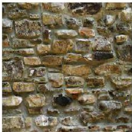
Example of walls
