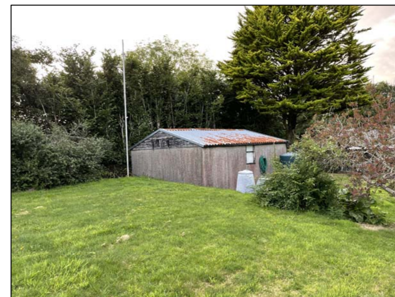
Rear View of Existing Garage
