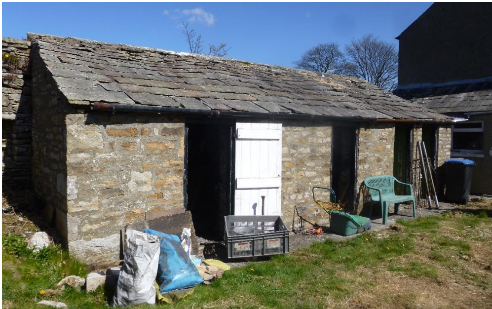
Fig 9: Existing stone outbuildings (stores and outside WC's) to northwest of site.
