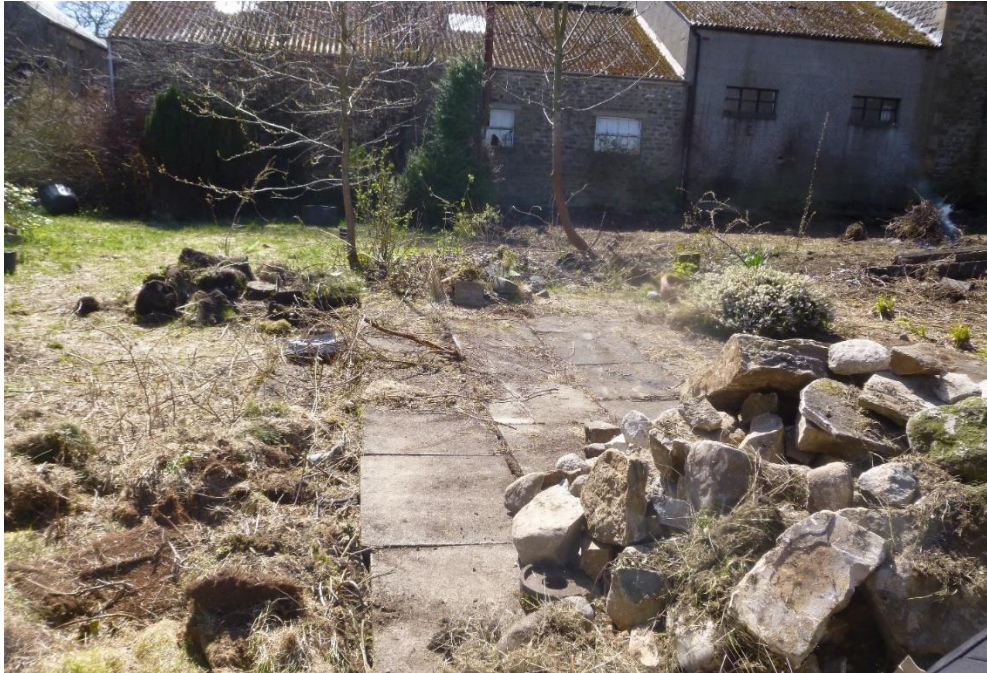
Fig 14: Existing site landscaping – modern concrete paving slabs. Industrial units behind.
