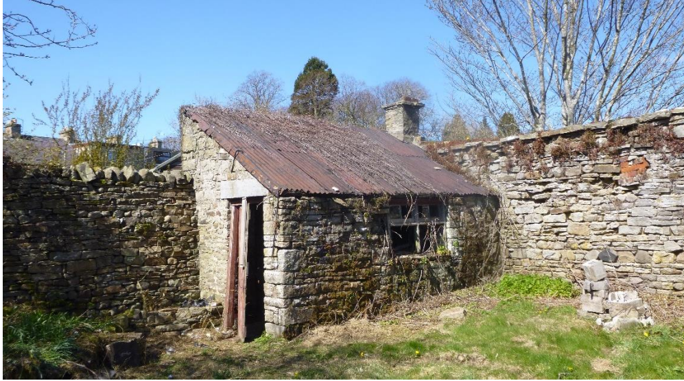
Fig 8: Existing stone outbuildings (washhouse) to northwest of site.
