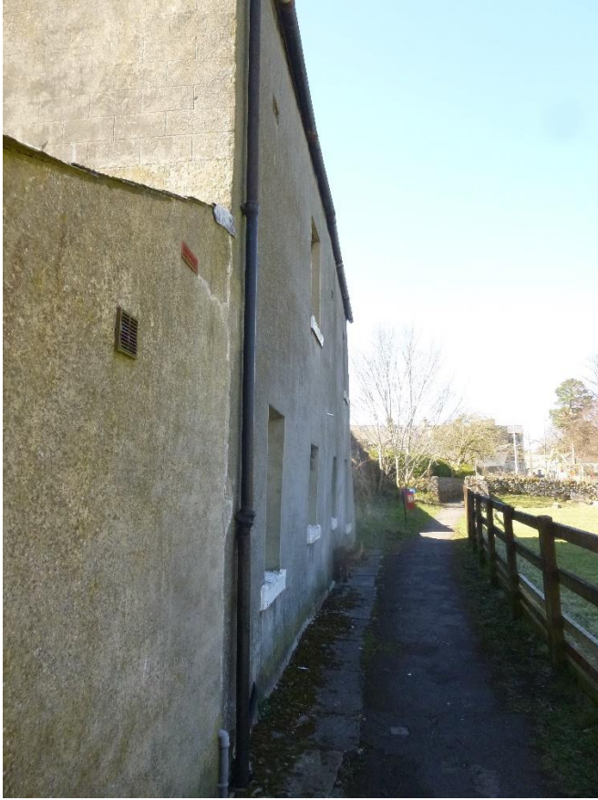
Fig 3: View to the north of Nelson Row, showing Public Footpath and field boundary to right of picture
