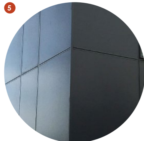
Grey cladding panels
