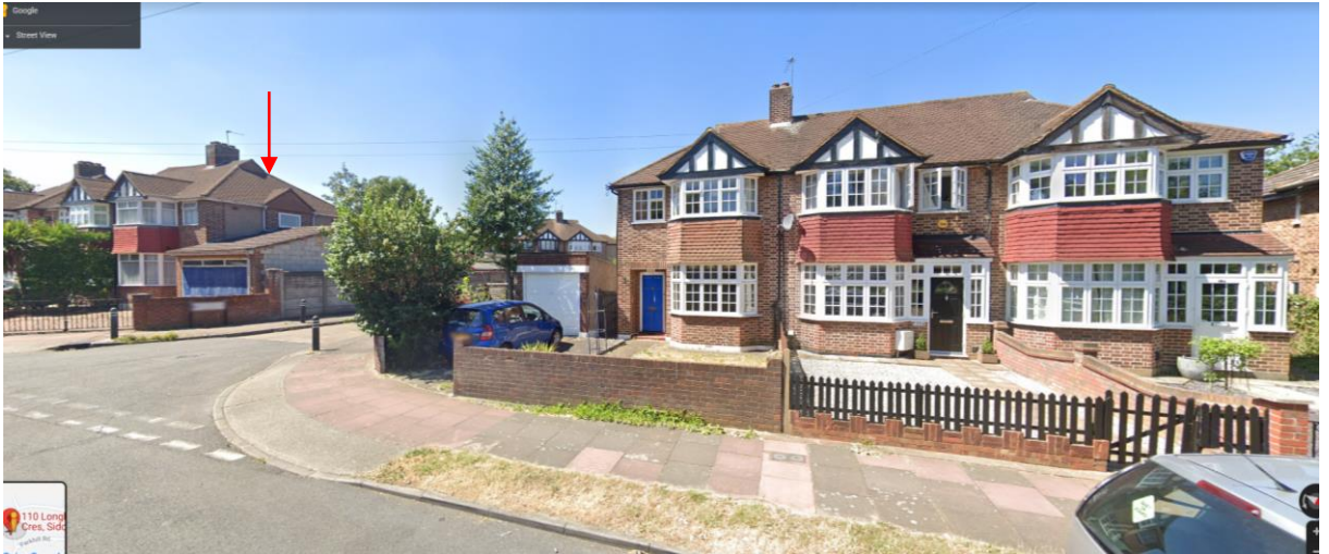
Image showing the existing street scene, similar terrace arrangement with a newly built dwelling to the side of pair of semi properties originally built exist and sets a precedent
