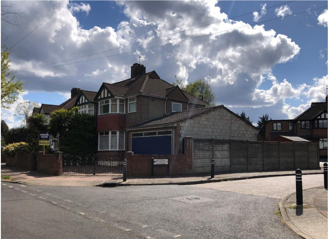
Photo showing existing front/side elevations
