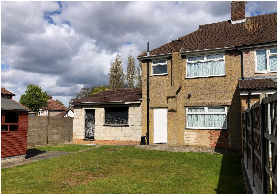
Photo showing existing rear elevation
