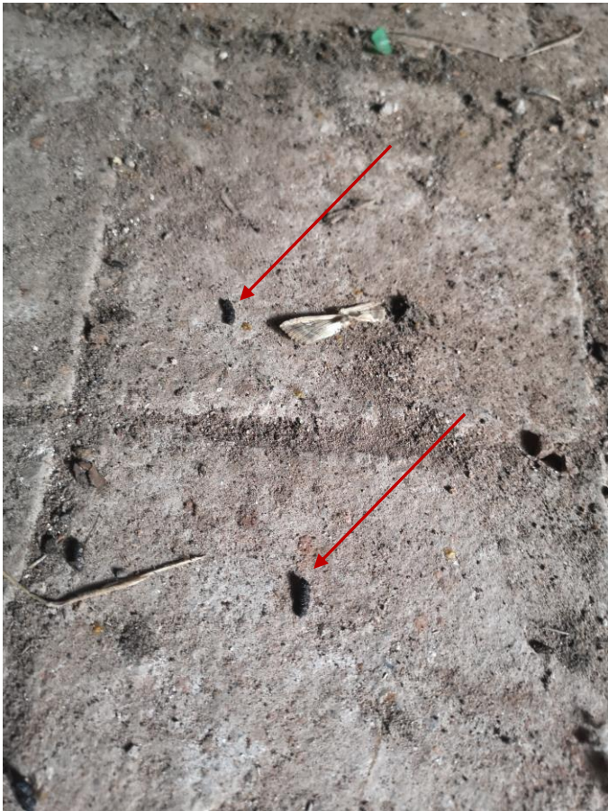
Figure 3 – droppings scattered within internal barn structure of B1.
