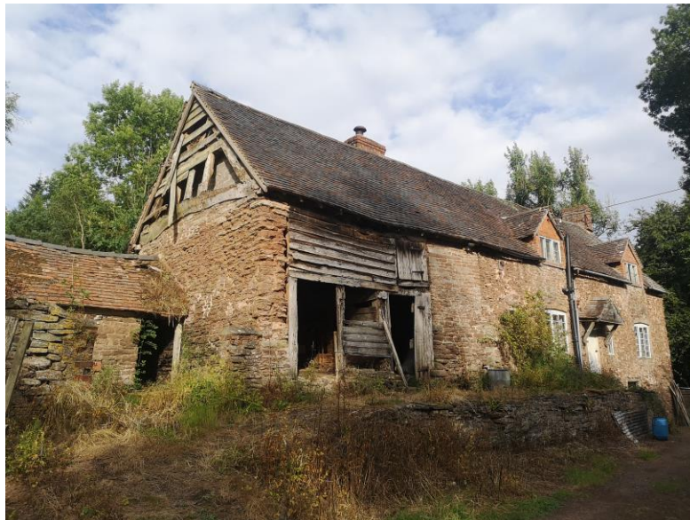
Figure 2 – north western aspect of B1
