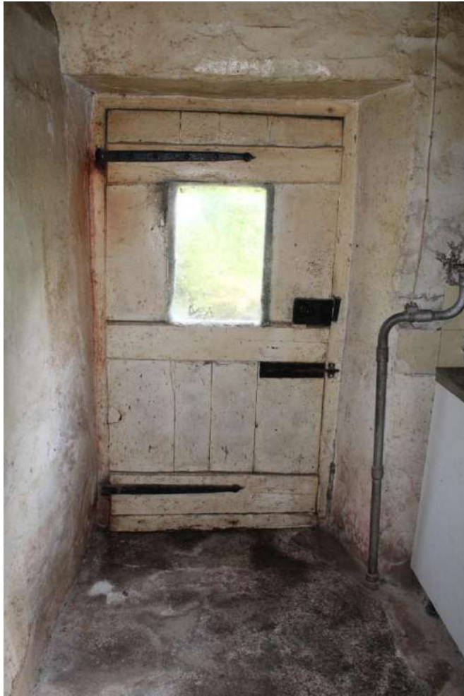
Photo 20: View northeast of rear doorway in central passage
