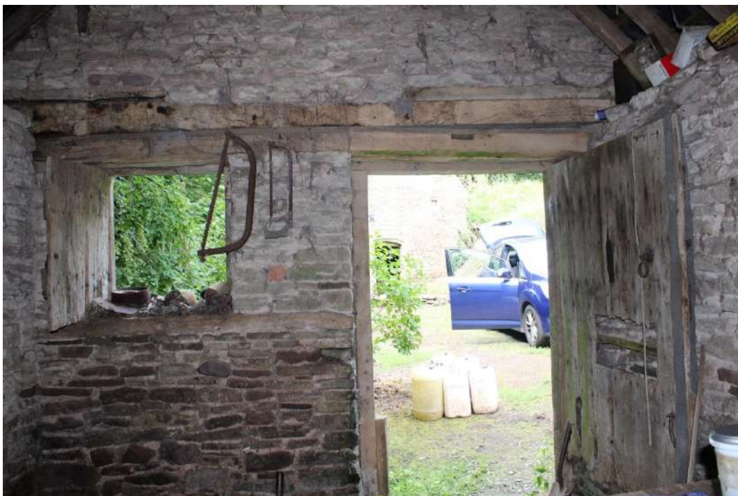
Photo 41: View northwest through northern room of Bakehouse towards Mill
