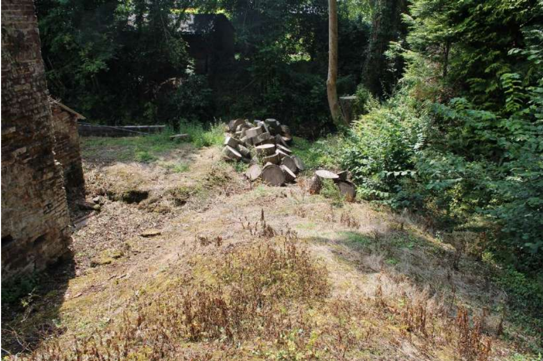
Phot 6: View southwest from mill pond with wheel pit to left and overflow channel to right leading to Clee Brook
