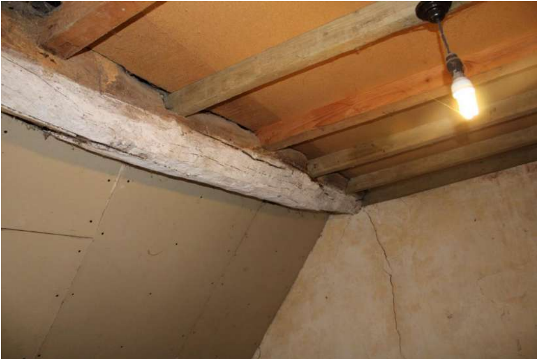
Photo 27: Ceiling in northern bedroom showing purlin
