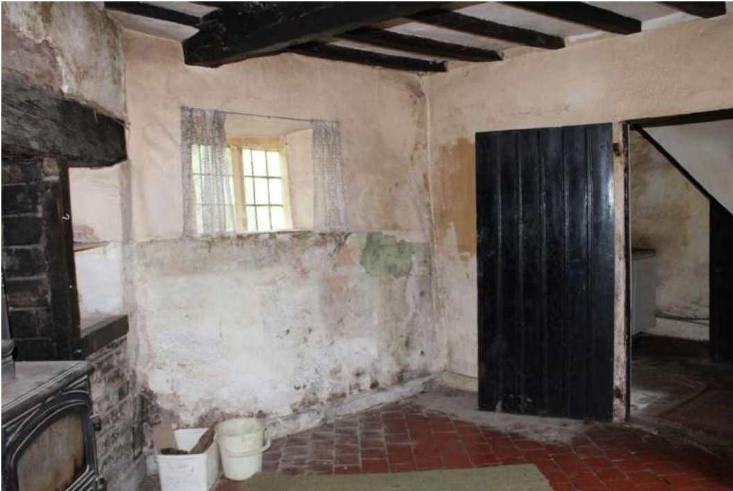
Photo 18: View southeast of northern ground floor room towards central passageway
