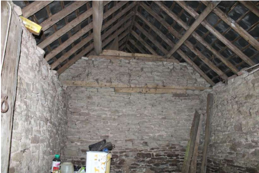
Photo 40: View southeast along northern room of Bakehouse
