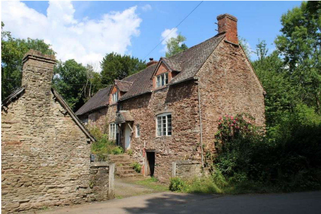
Photo 16: View north of southwestern façade of the Mill House with Bakehouse to the left
