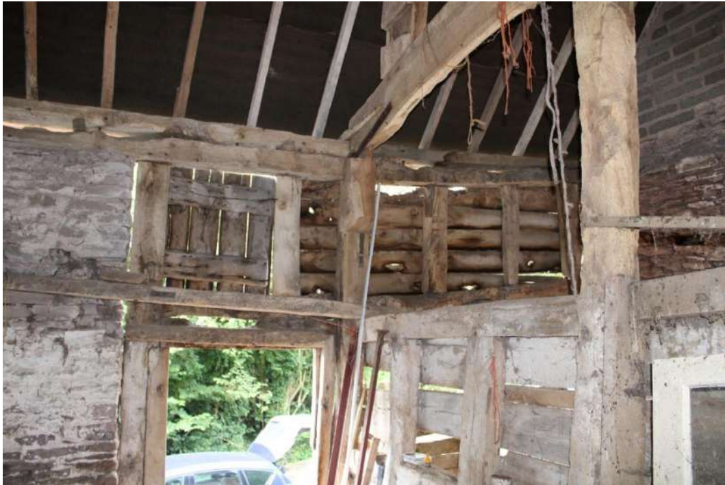
Photo 33: View southwest through barn showing timber infilled door
