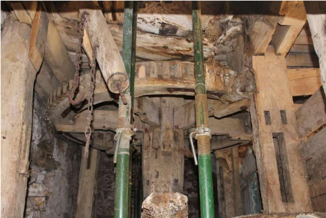
Photo 13: View from window in side of Mill showing part of surviving workings
