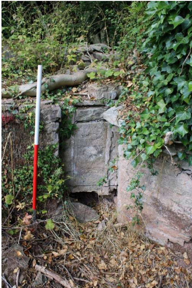
Photo 7: View west of impression of sluice gate in later concrete infill on northwestern edge of mill pond, forming the overflow
