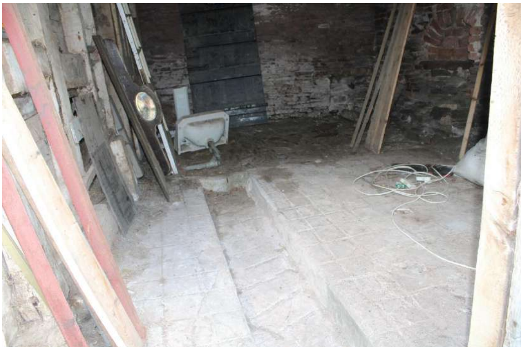
Photo 34: Floor of northern barn showing mx of bricks with drain and surviving cobbled area beyond
