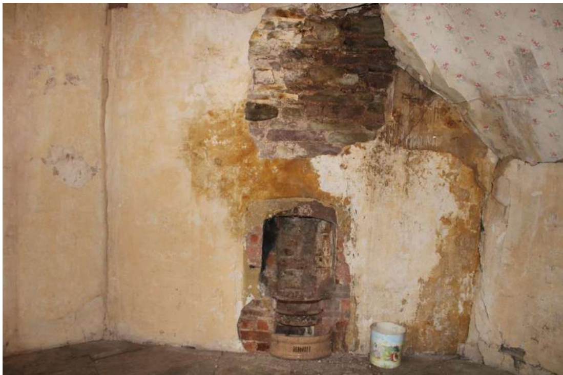
Photo 26: Fireplace in northeastern corner of room in northern bedroom
