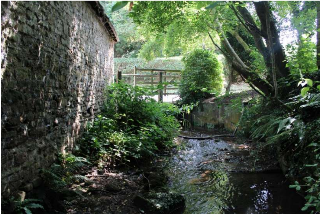
Photo 38: View southeast along southern side of the Bakehouse showing the Clee Brook running to and below the road
