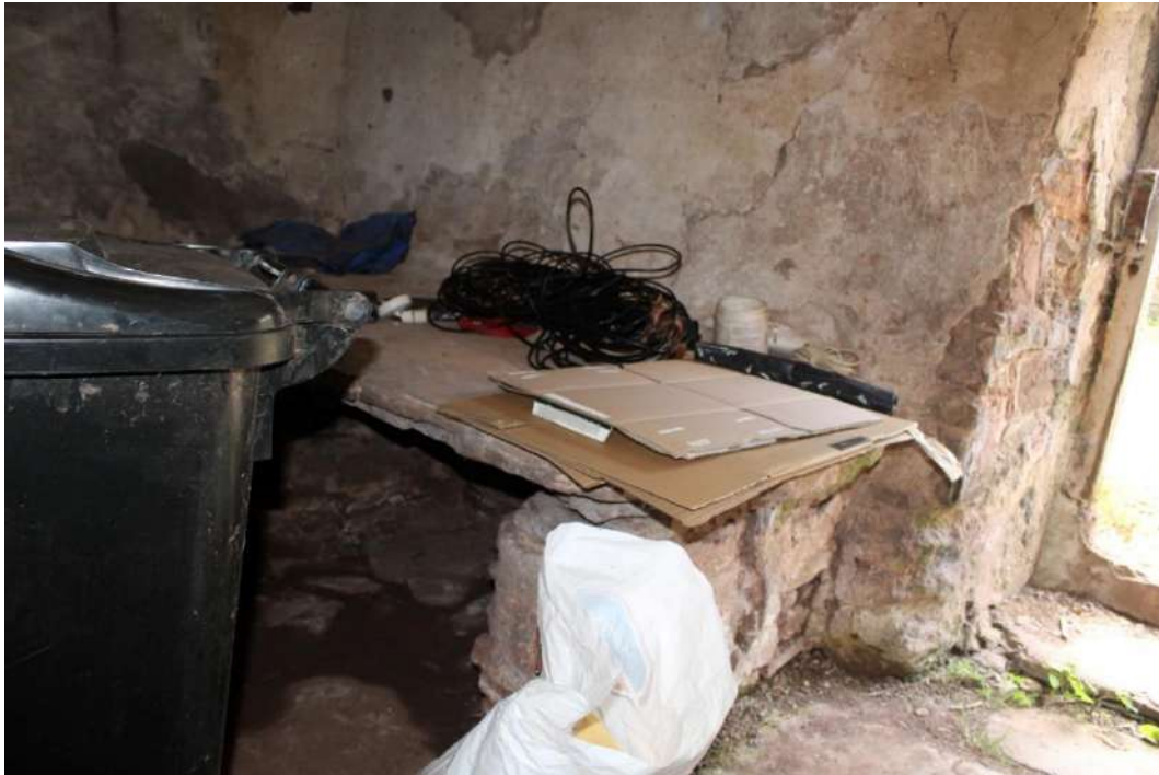
Photo 31: View southeast across basement showing stone slab bench adjacent to doorway
