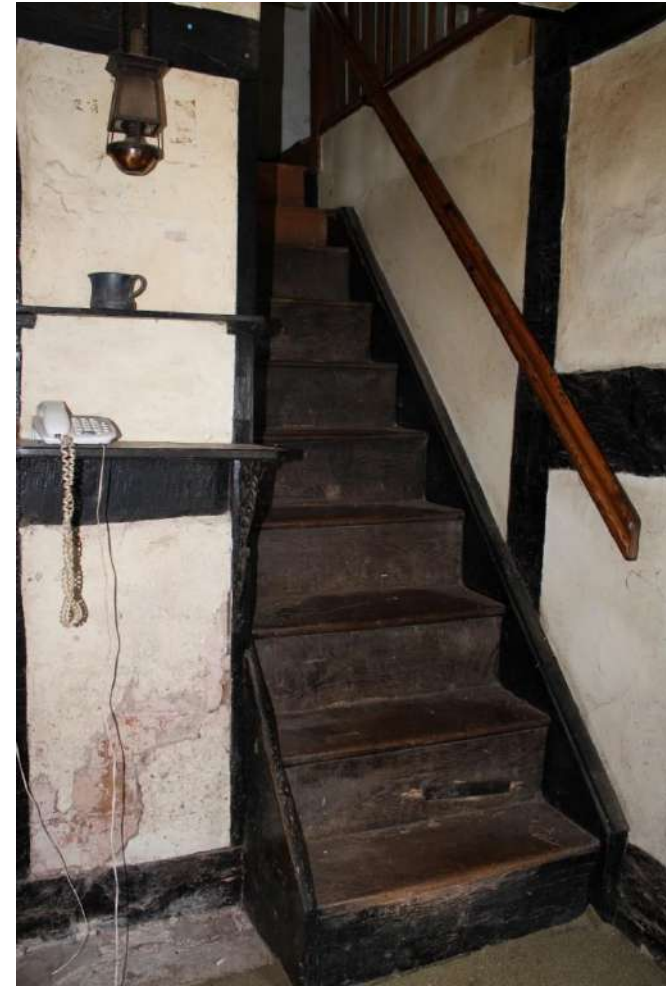
Photo 23: View east of stair in central passage
