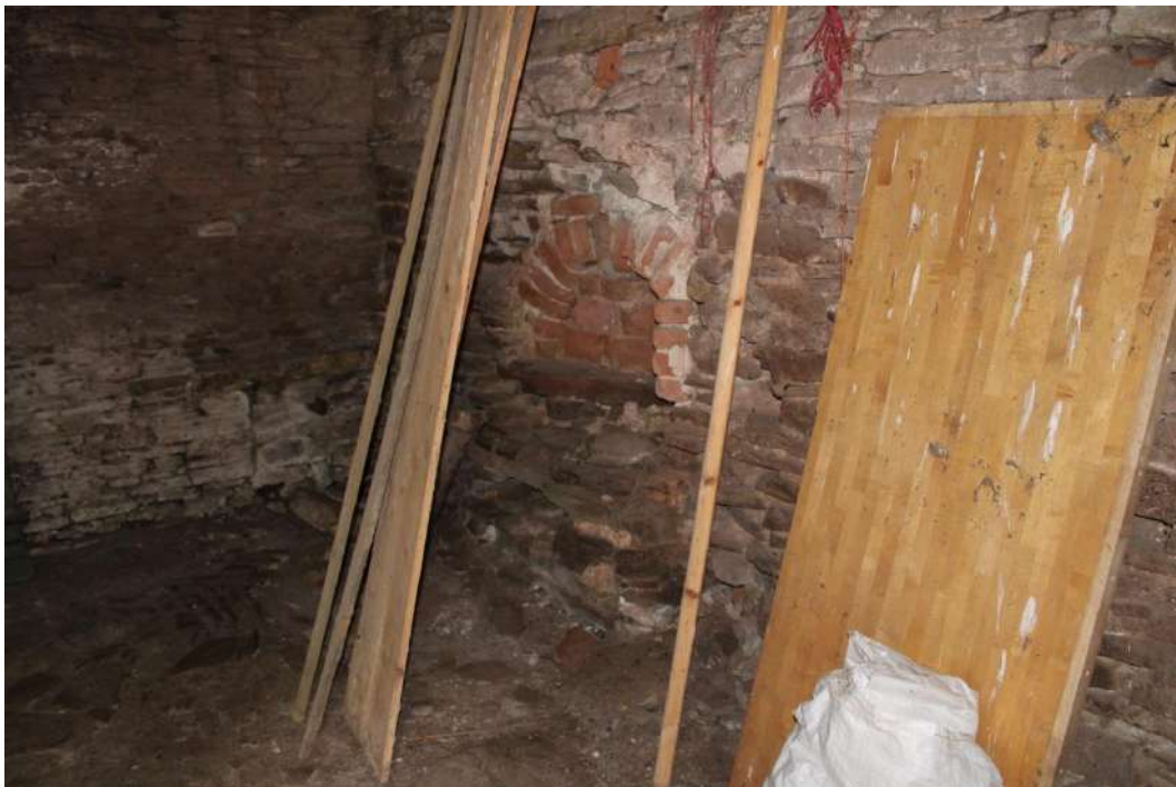
Photo 36: View into southeastern corner of barn showing brick arch adjacent to location of large fireplace within Mill House
