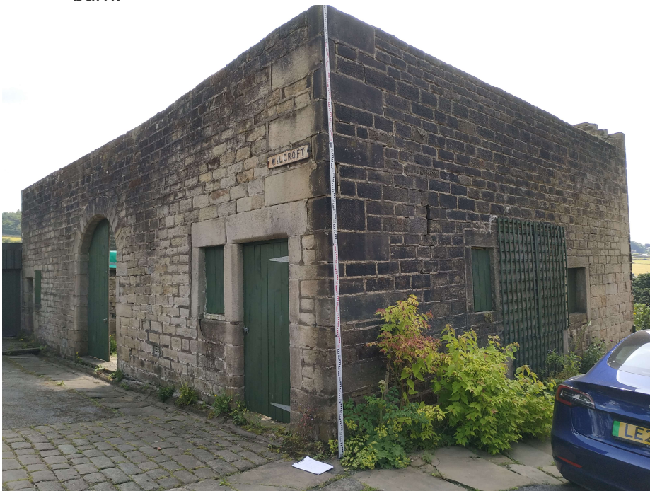
P5 Wilcroft Barn, north and west sides
