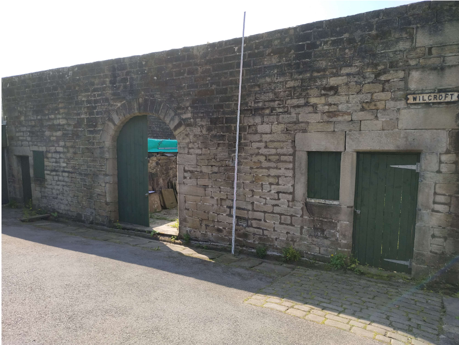
P4 Wilcroft Barn, north side
