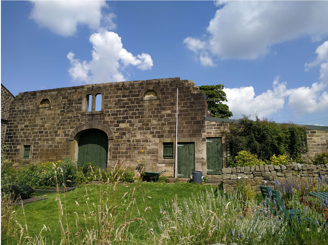
P6 Wilcroft Barn, south side
