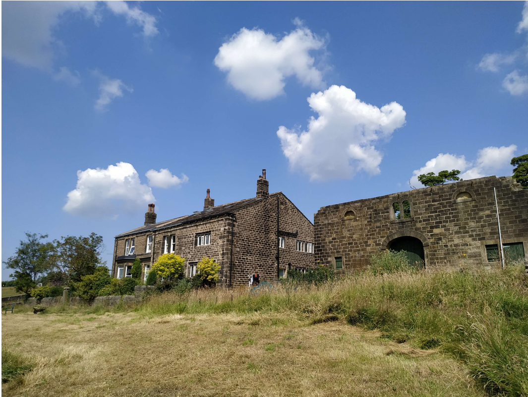
P1 Wilcroft House (left), Wilcroft Farmhouse and Barn viewed from south 05.08.2021
