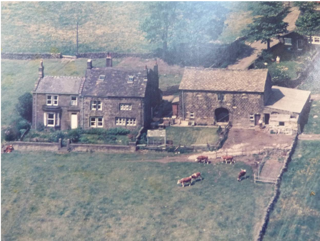
P2 Aerial view of Wilcroft House, Wilcroft Farmhouse and Wilcroft Barn (1982)
