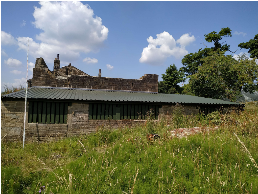
P7 Wilcroft Barn, east side
