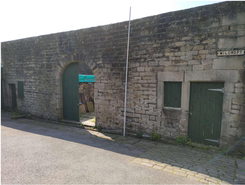
P4 Wilcroft Barn, north side
