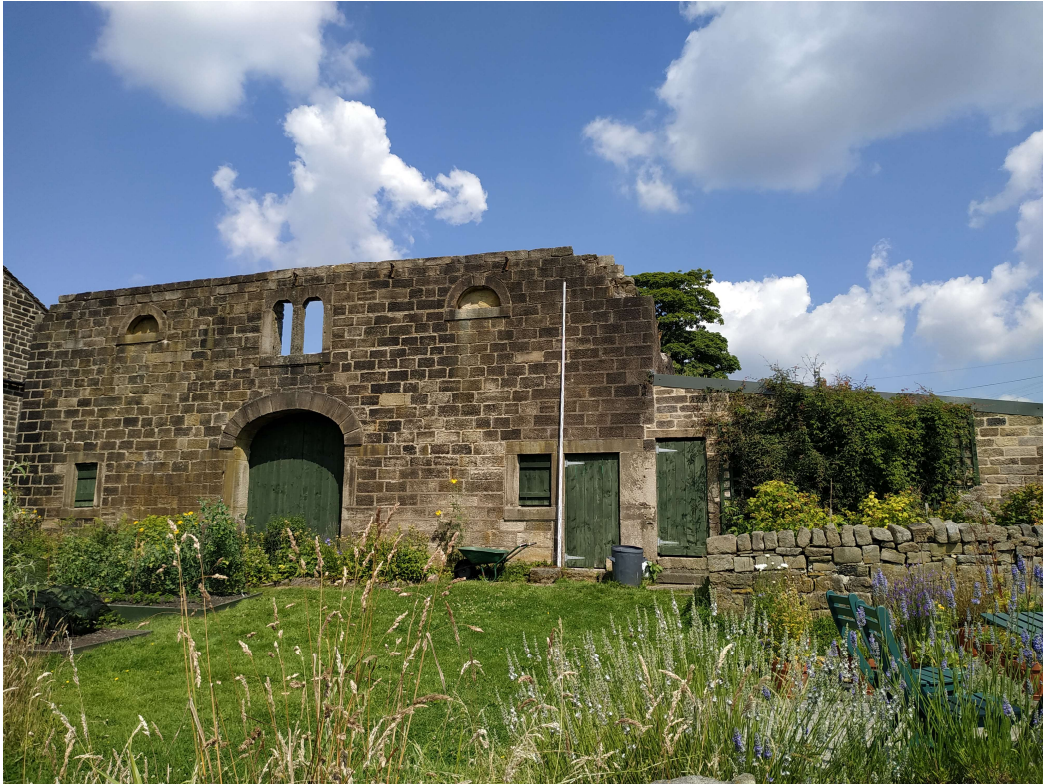
P6 Wilcroft Barn, south side
