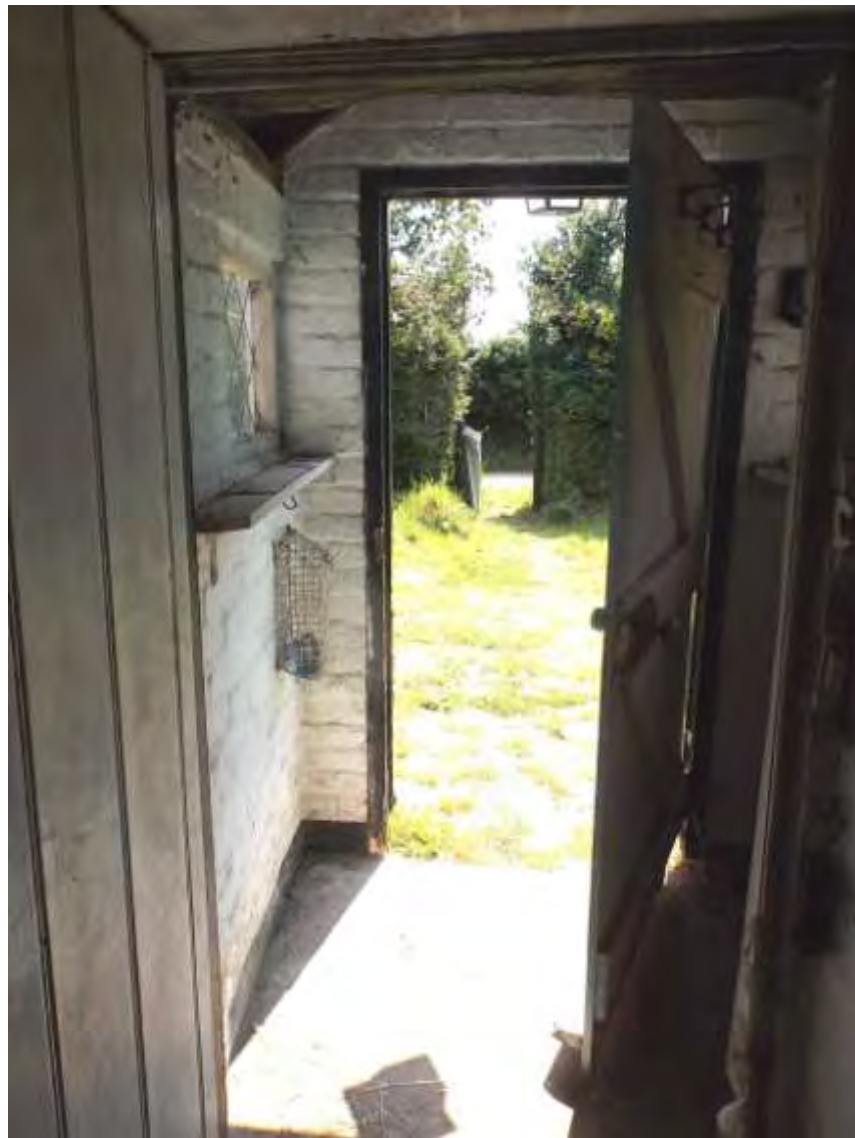
Fig 4.1; Porch from living room
