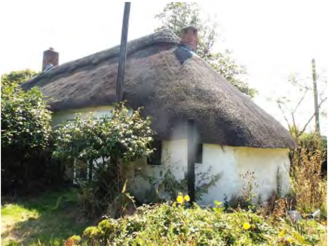
Fig 3.4.12; West end from northwest
