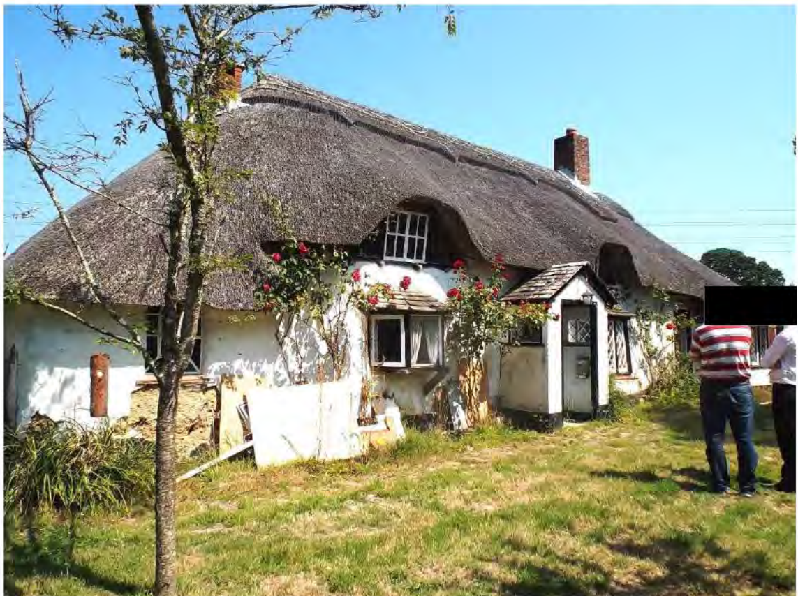
Fig 2.2; House from southwest
