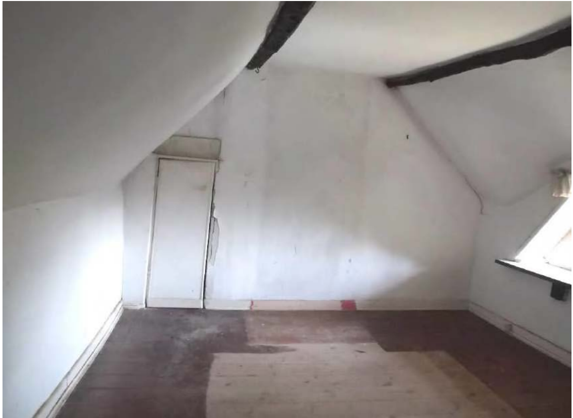
Fig 4.9; Bedroom looking from head of stairs
