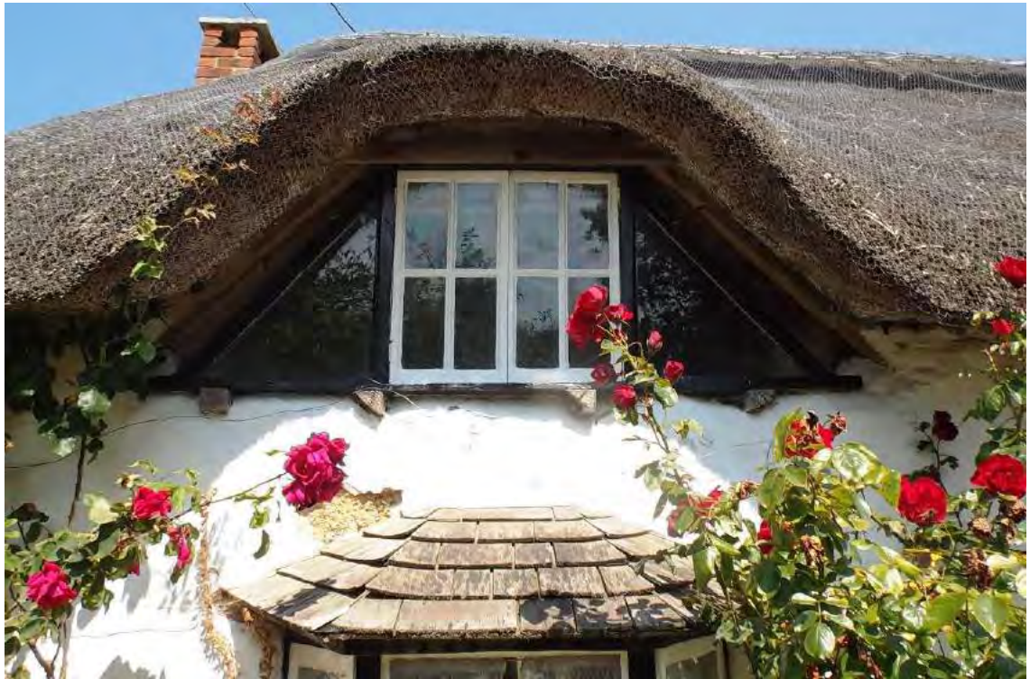
Fig 3.5.12; West eyebrow window over shingle roof to kitchen oriel window
