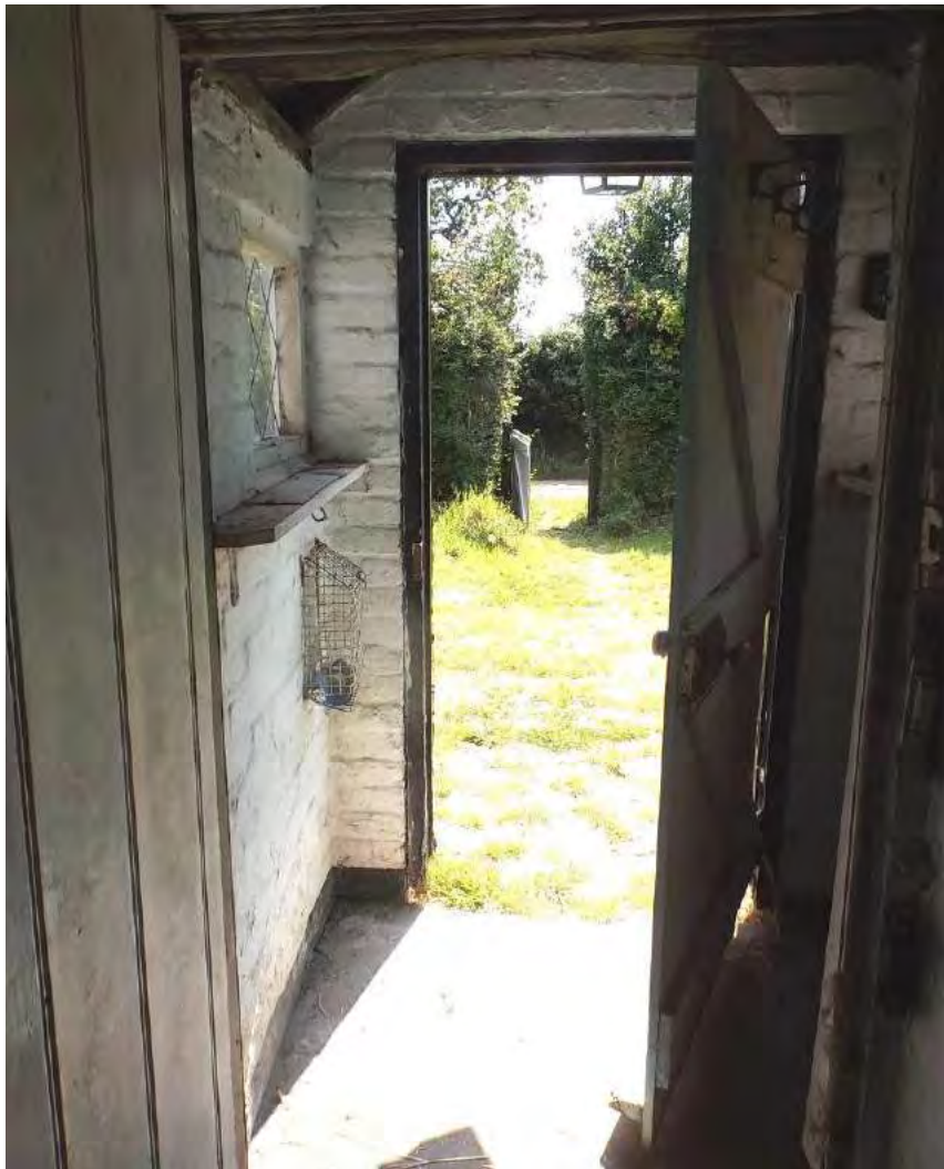
Fig 4.1; Porch from living room
