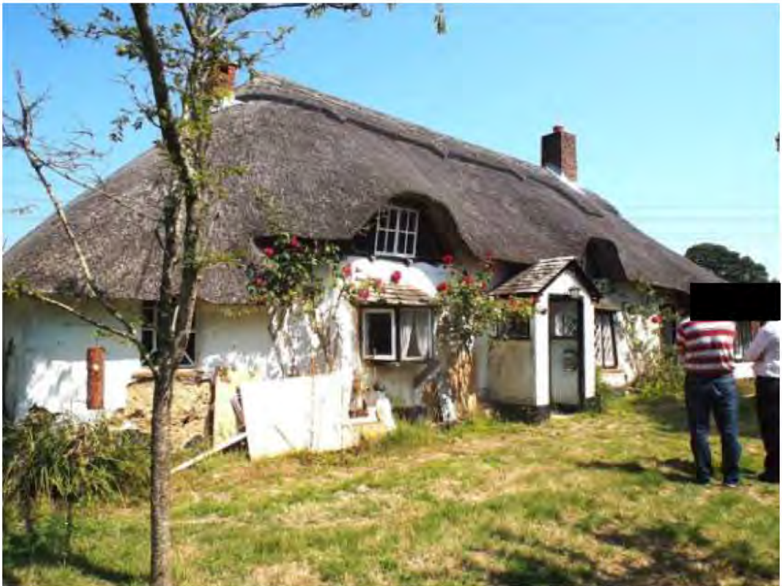
Fig 2.2; House from southwest
