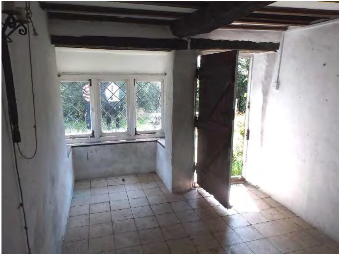
Fig 4.10; East extension room looking from rear to front
