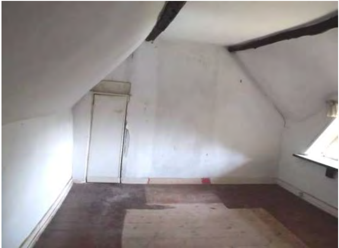
Fig 4.9; Bedroom looking from head of stairs
