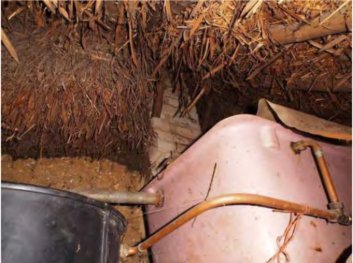
Fig 4.11.2; West extension roof structure and original half hip to main house
