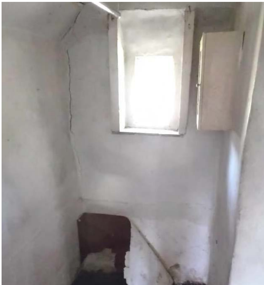
Fig 4.4; Lobby in northwest
