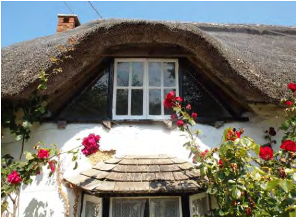
Fig 3.5.12; West eyebrow window over shingle roof to kitchen oriel window
