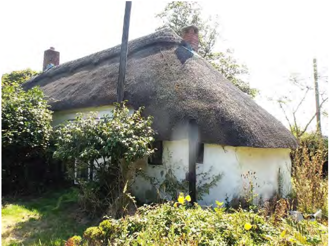
Fig 3.4; West end from northwest
