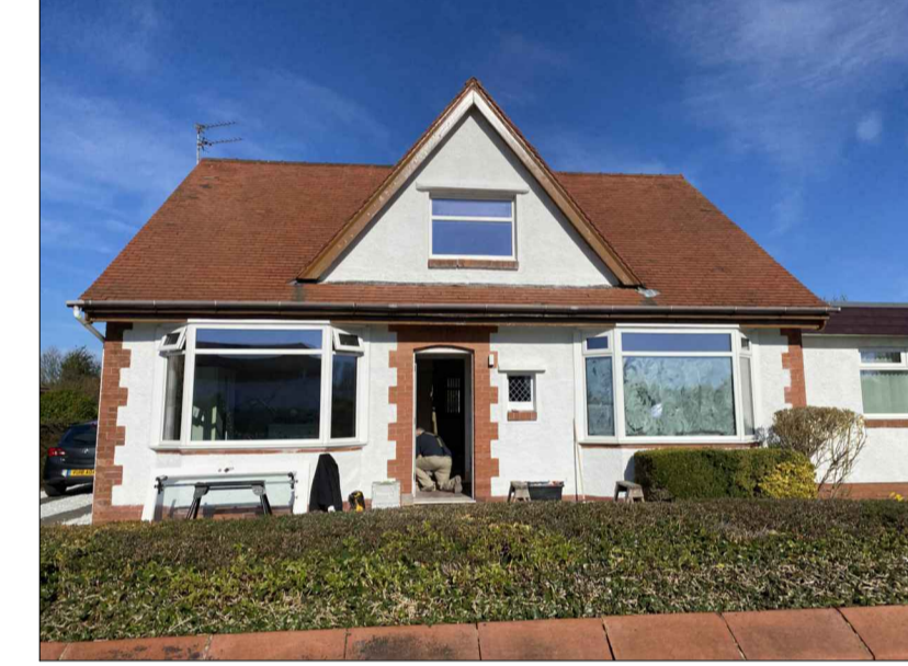
05 Existing Photos Scale NTS @ A1
